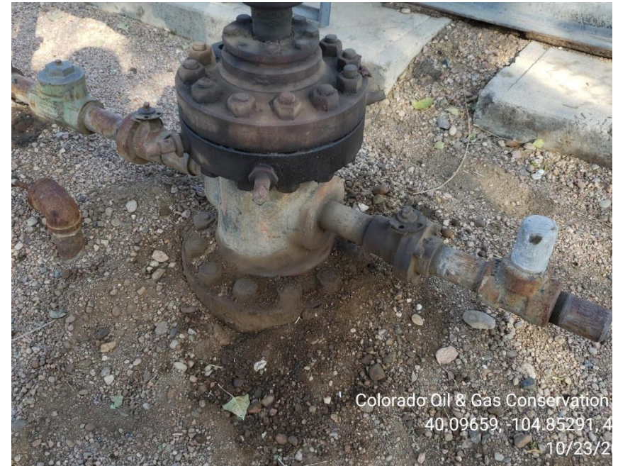
Photo #2 Stained soil around WH
