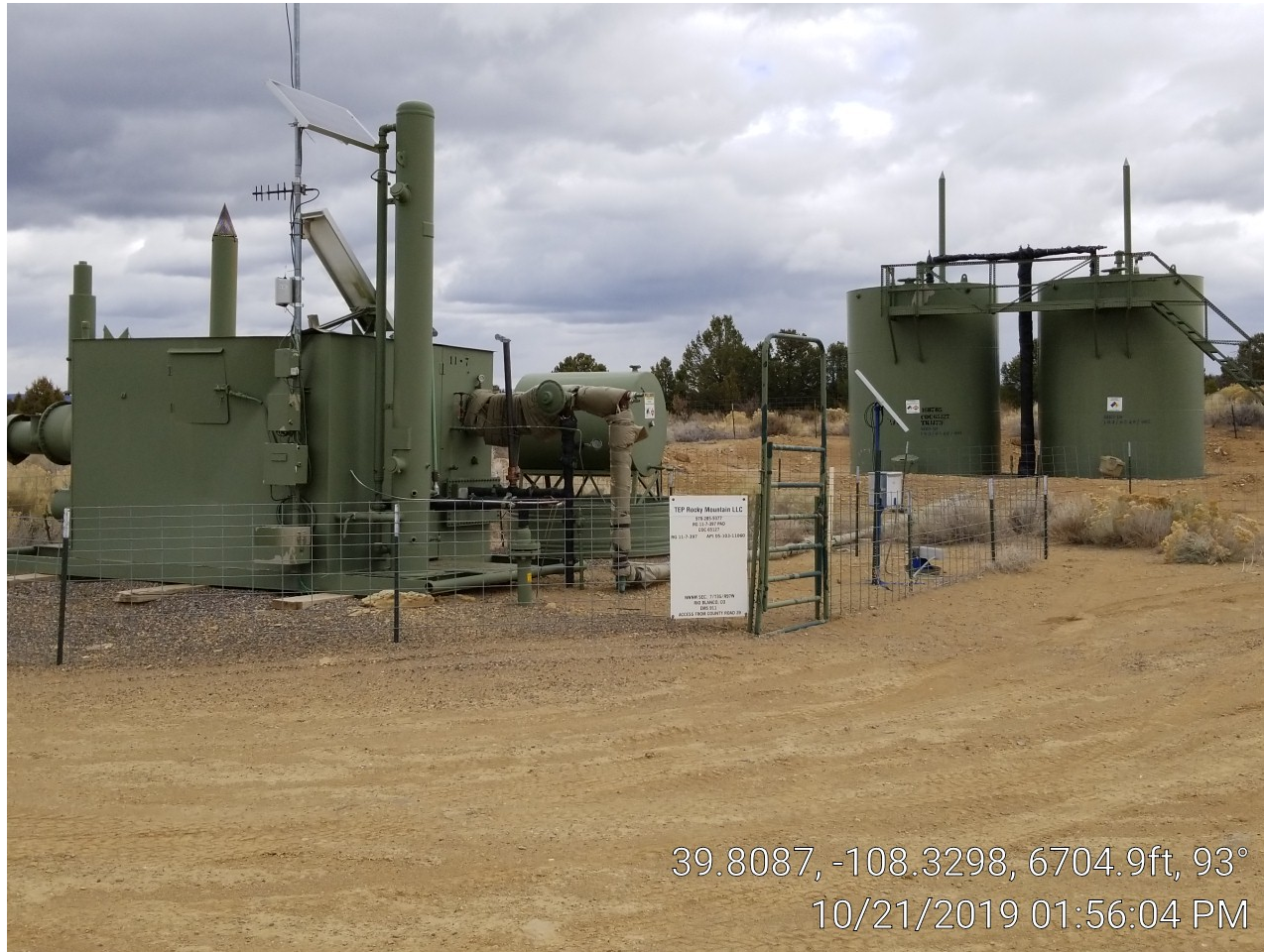
Photo 2. Separator & tanks.
