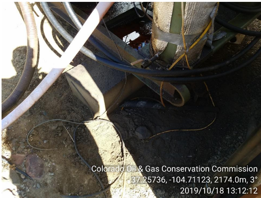
PHOTO 3: AREA OF IMPACTED SOIL AROUND AND UNDER ENGINE SKID. Properly treat or dispose of oily waste in accordance with 907.e. CA DATE 11-18-19
