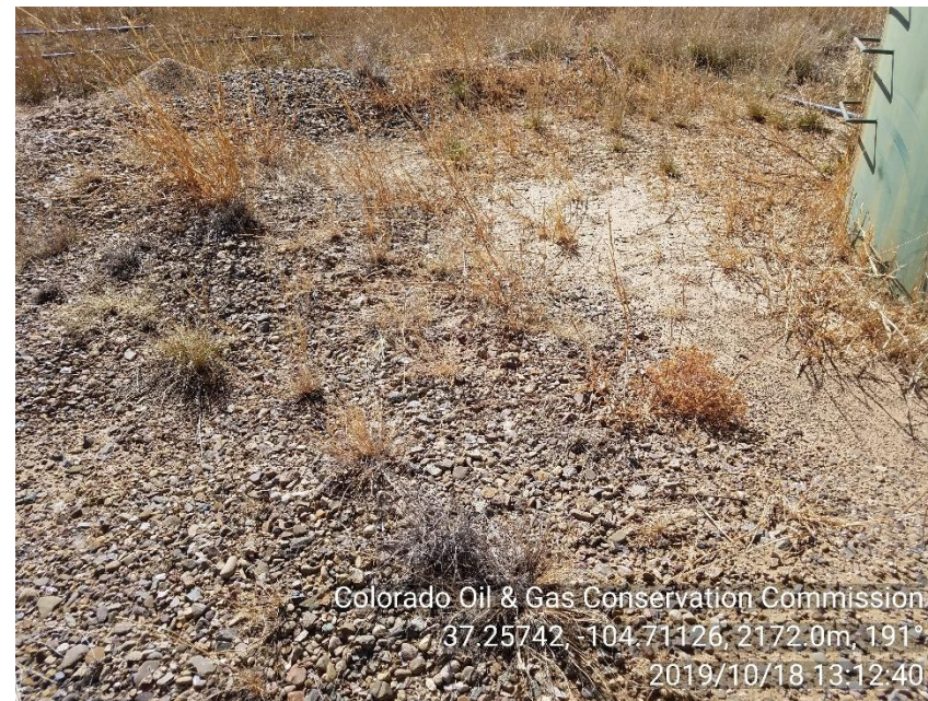
PHOTO 4: CONTAINMENT BURMS AROUND PRODUCED WATER TANK IS IN ADEQUATE FOR PROPER CONTAINMENT. Repair or install berms or other secondary containment devices per Rule 906.d.(1). CA DATE 11-18-19
