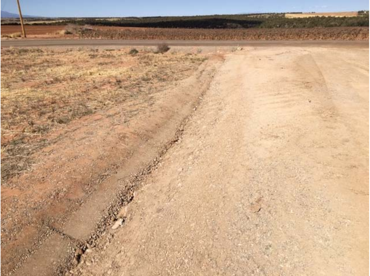
Drainage swale constructed on west side of access road at the CB-3 location.
