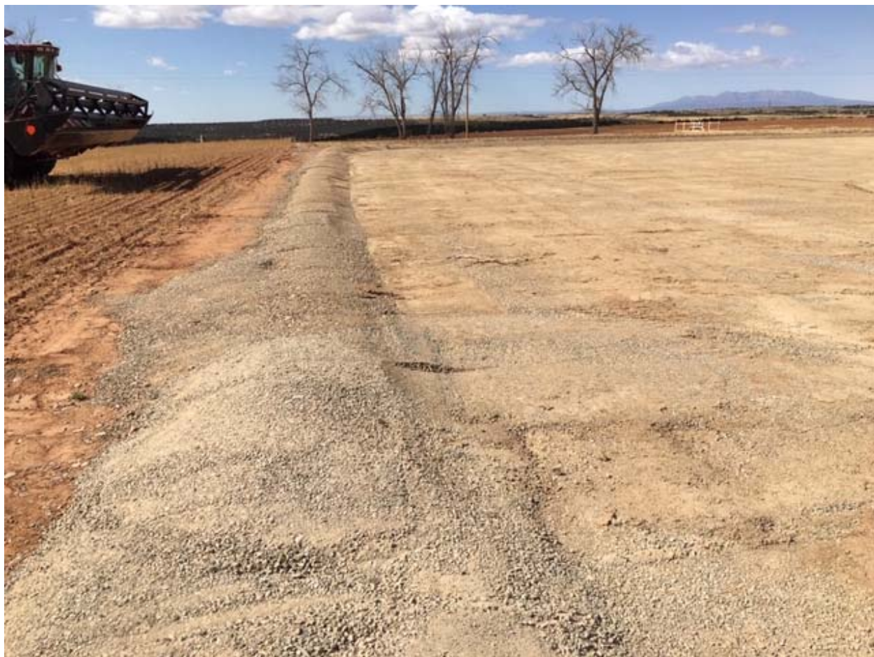
Gravel berm constructed on south side of well pad at the CB-3 location.
