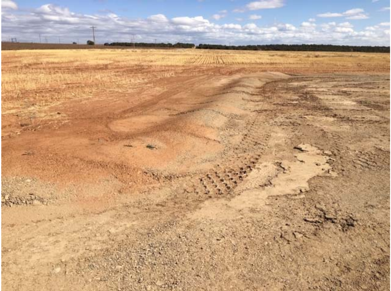
Gravel berm constructed on northeast side of well pad at the CB-3 location.
