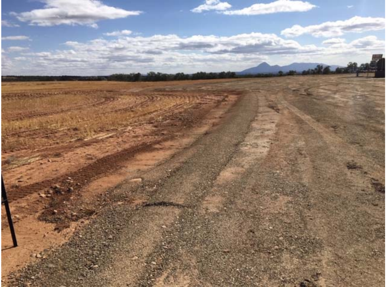
Gravel berm constructed on east side of access road at the CB-3 location.
