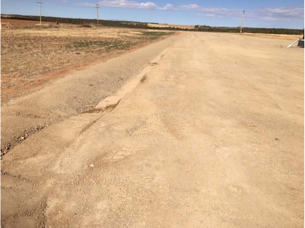
Gravel berm constructed on south half of west side of well pad at the CB-3 location.
