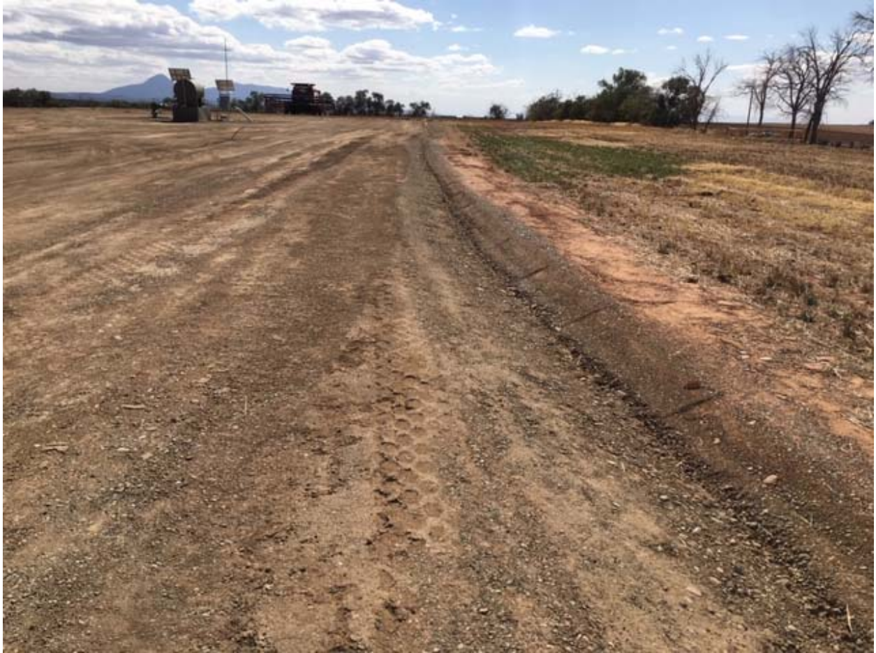
Drainage swale constructed on north half of west side of well pad at the CB-3 location.
