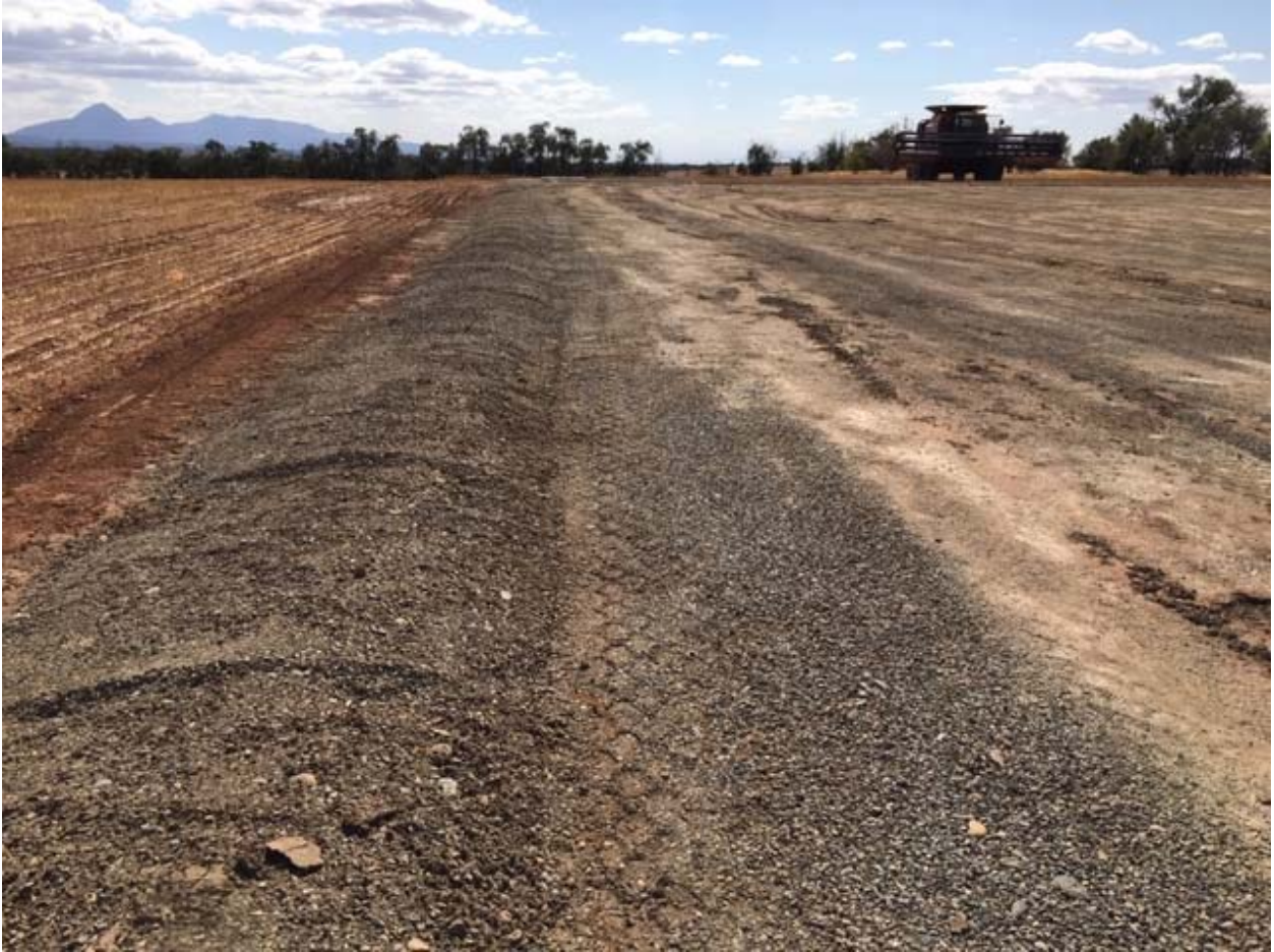
Gravel berm constructed on east side of well pad at the CB-3 location.
