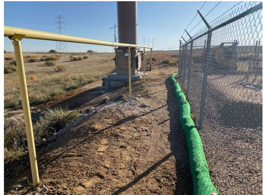
Photo NBL3. Filtrexx installed outside fence. Erosion repaired, and sloped compacted and tracked.
