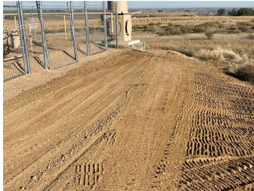
Photo NBL1. Erosion back-filled, and slopes compacted and tracked.
