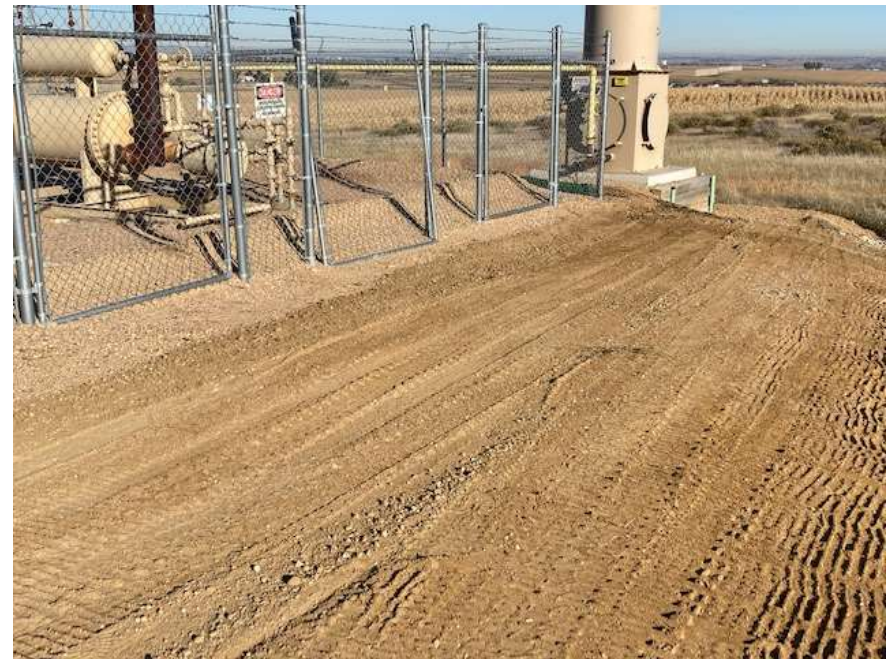
Photo NBL2. Erosion back-filled, and slopes compacted and tracked.
