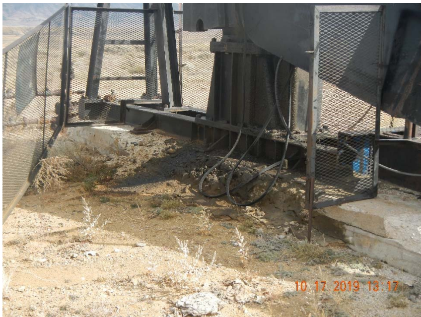
Photo 2. Stained soil at pump jack base.
