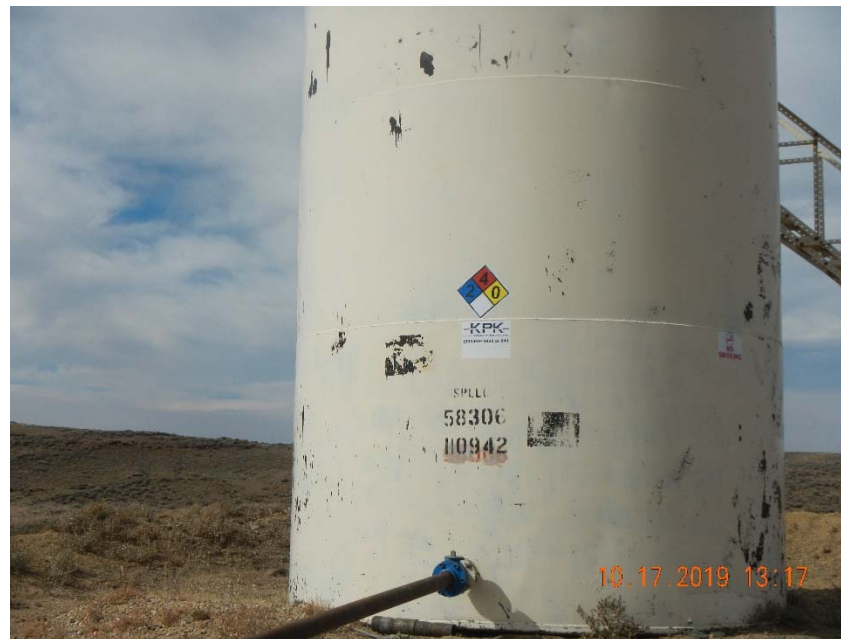
Photo 3. Incomplete tank label; no contents, no capacity.
