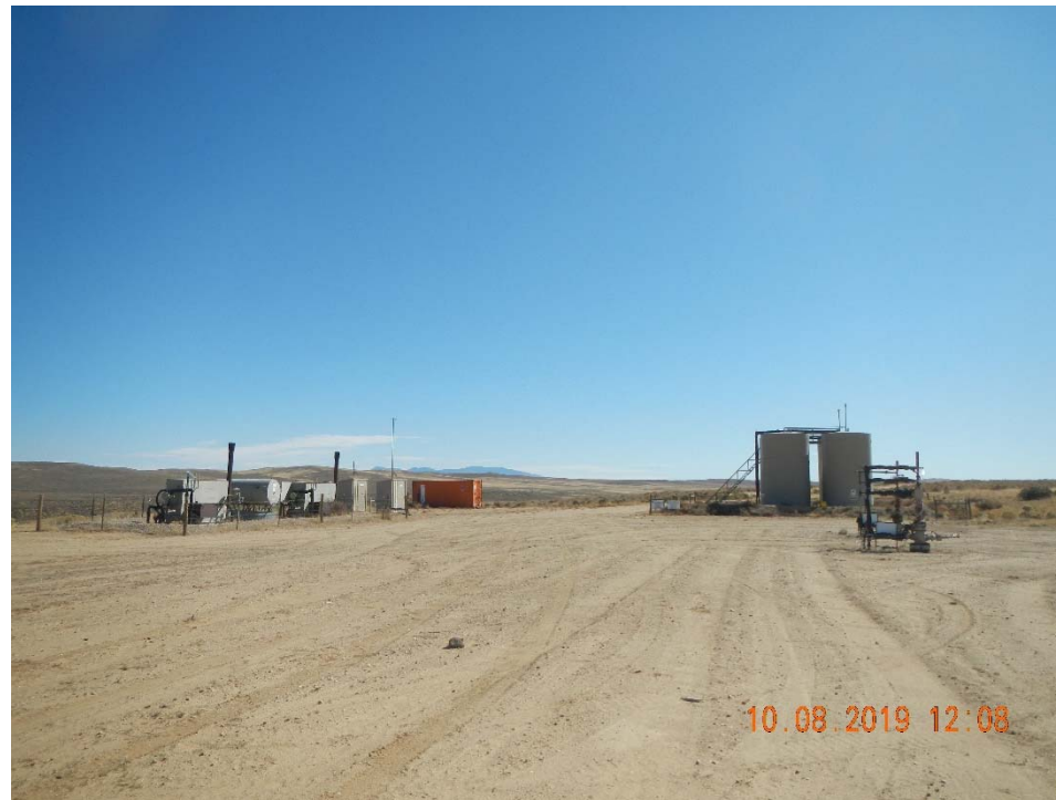
Photo 1. Overview of location taken facing southeast.
