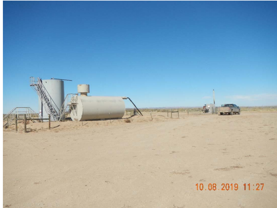
Photo 1. Overview of location taken facing northwest.
