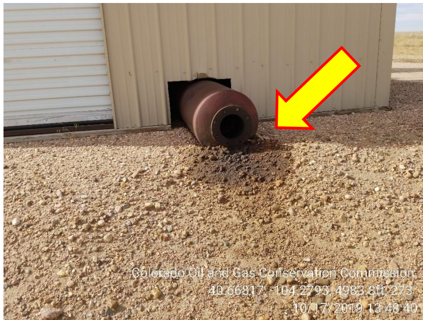
Photo 7 – Stained Soil at Exhaust
