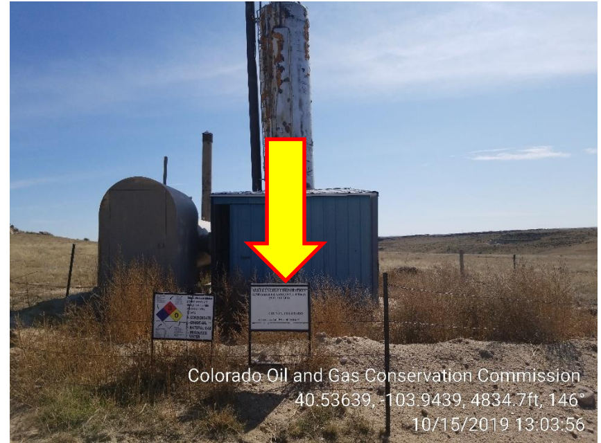
Photo 4 – Weeds at Heater Treater/Separator. Sign has faded no longer legible.
