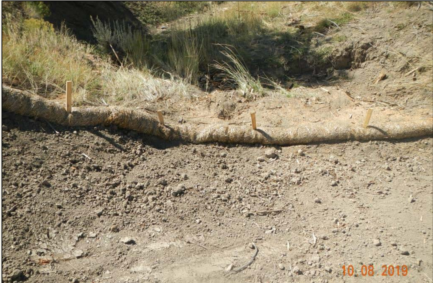
Photo 8. View of wattle down-slope of Photo 6 across stream bed. This is not an appropriate stormwater BMP in this area as it is inadequate and improperly installed (not trenched), as evidenced by flow patterns beneath the wattle.
