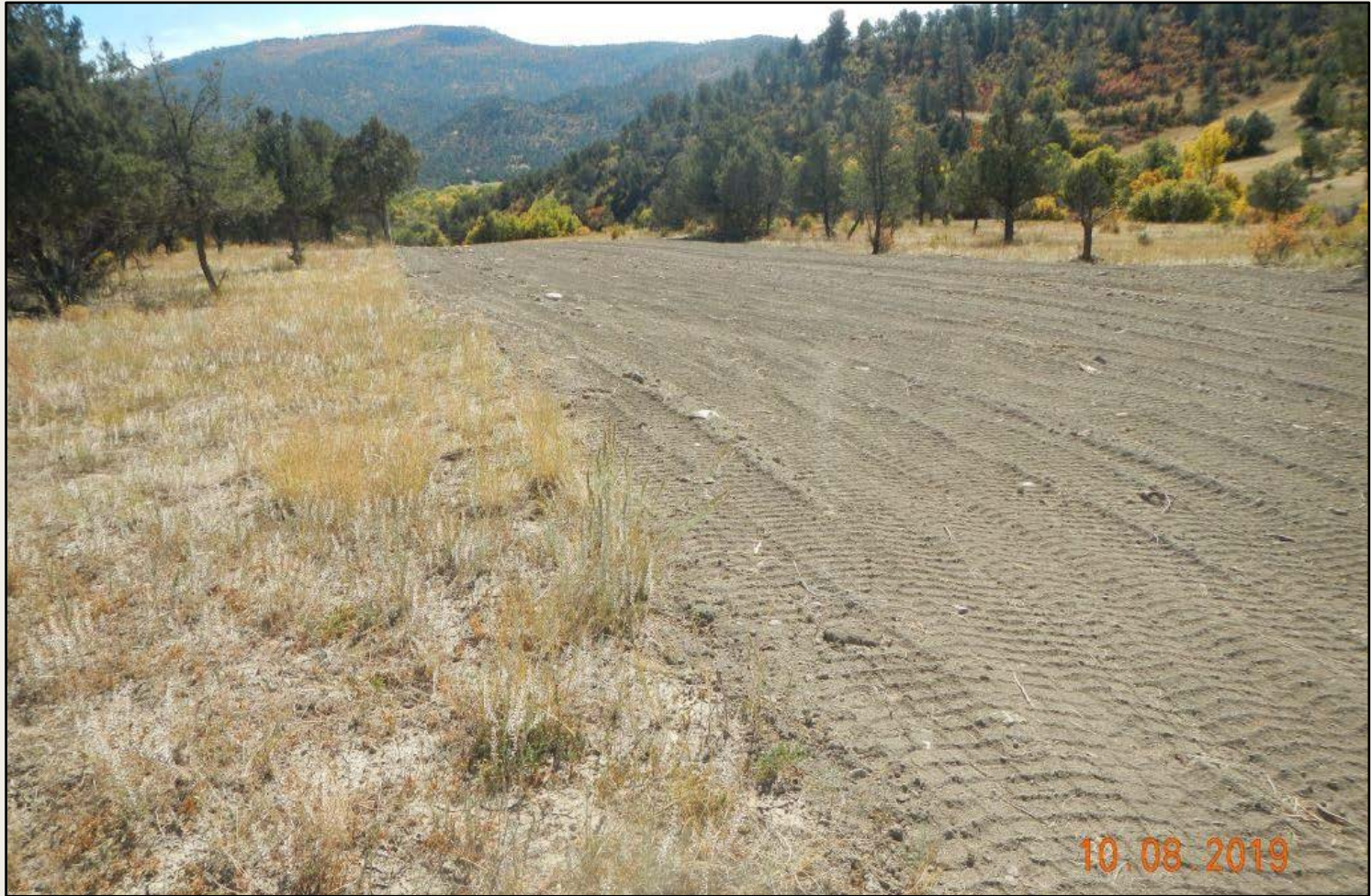
Photo 6. View of pipeline right of way that is not stabilized.
