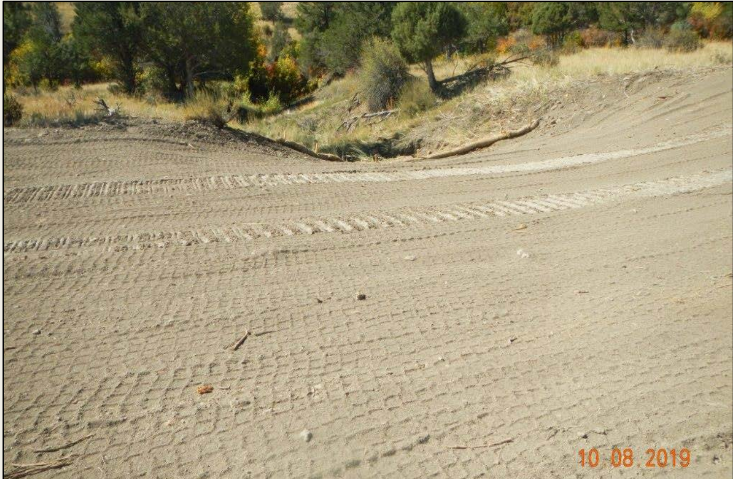
Photo 7. View of another portion of the pipeline right of way, showing bare soils over portion where right of way crosses stream and no insufficient stormwater controls are in place.
