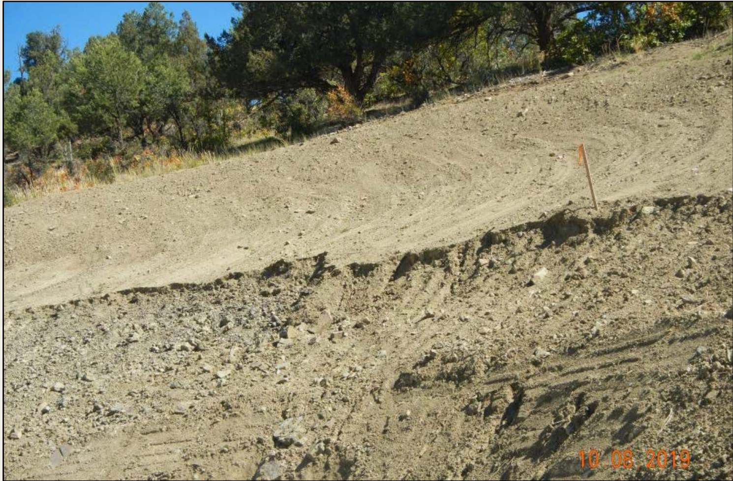
Photo 3. View of the eastern cut-slope facing upslope. Bare soils are not stabilized. Steep slopes will likely need to be reduced for successful revegetation.
