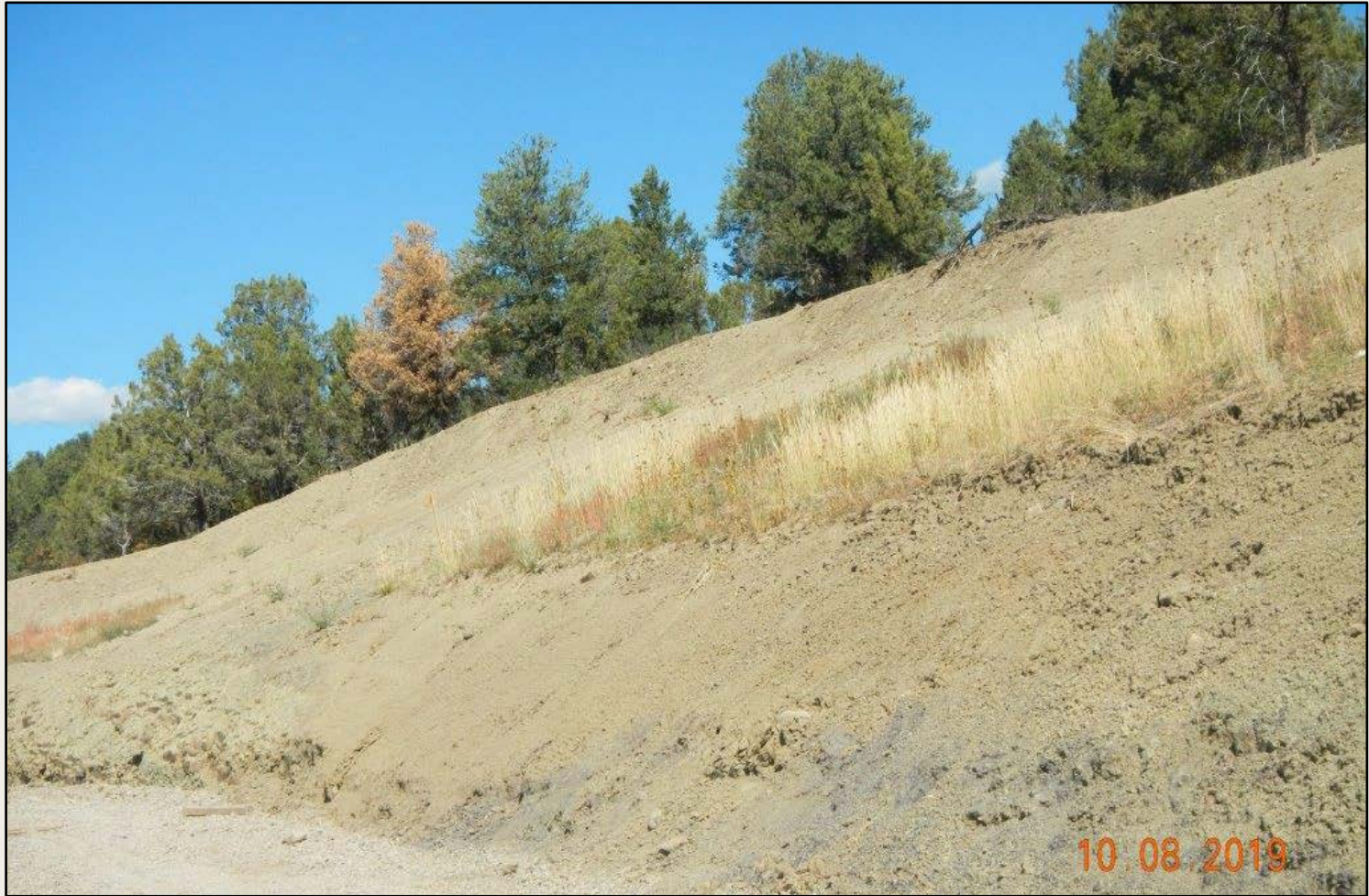
Photo 4. Another view of the eastern cut-slope. Bare soils are not stabilized.
