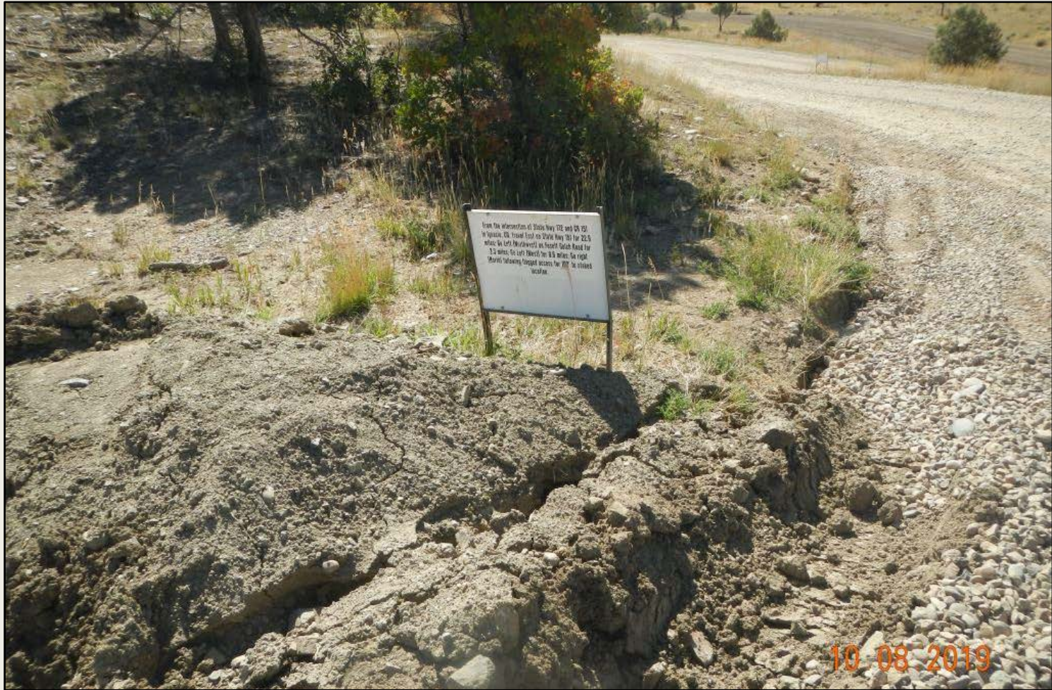
Photo 5. View of erosional channels forming and sedimentation along the access road, at the well pad entrance.
