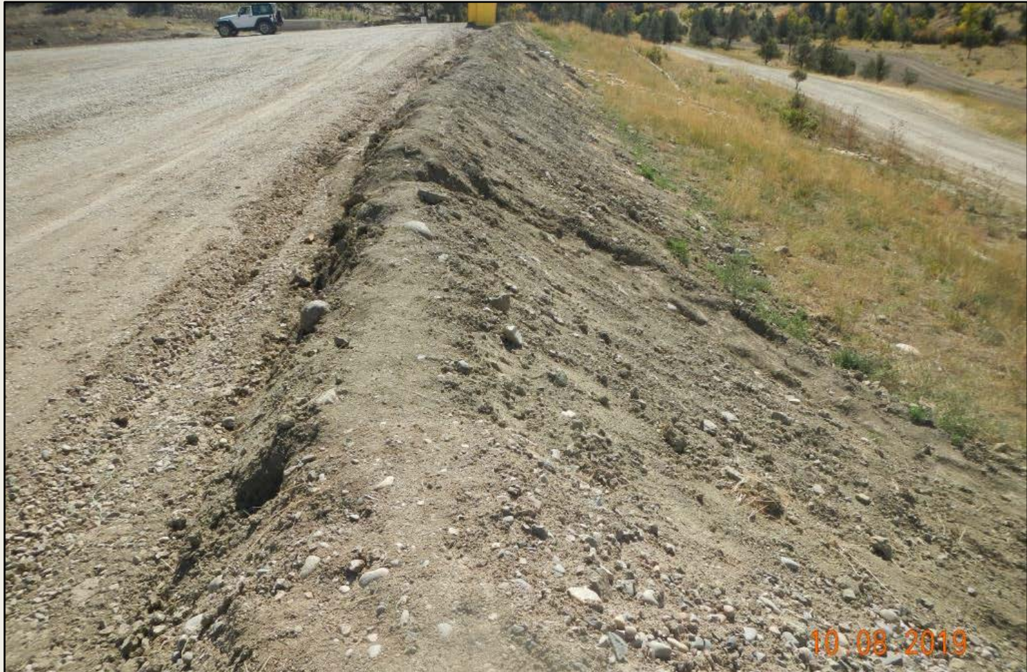
Photo 2. View of the western cut-slope from the northwestern corner facing southward. Bare soils on slope need stabilization.
