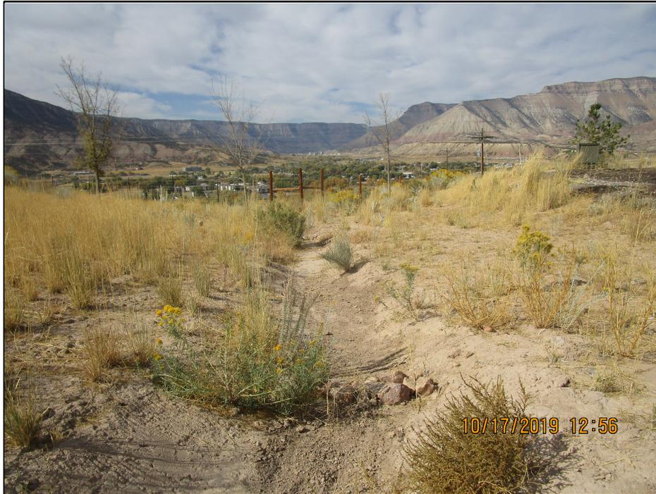
rilling and "sediment migration" along the north west corner has been raked, seeded and mulched.
