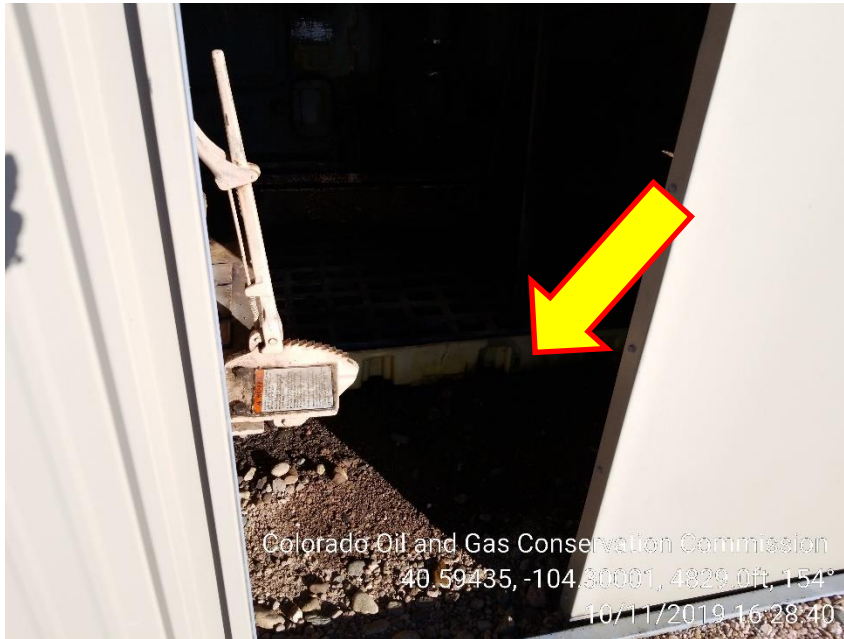
Photo 5 – Stained Soil at Engine
