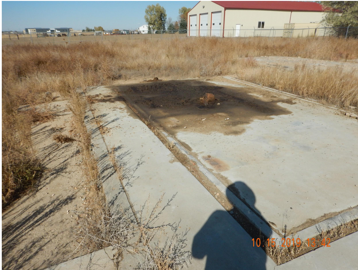
Photo 3. Photo taken from inside the southern compressor station, facing North. Photo illustrates the Operator has failed to perform final reclamation activities (i.e, concrete pad remains). Operator shall comply with the Environmental staff corrective actions regarding the oily material.
