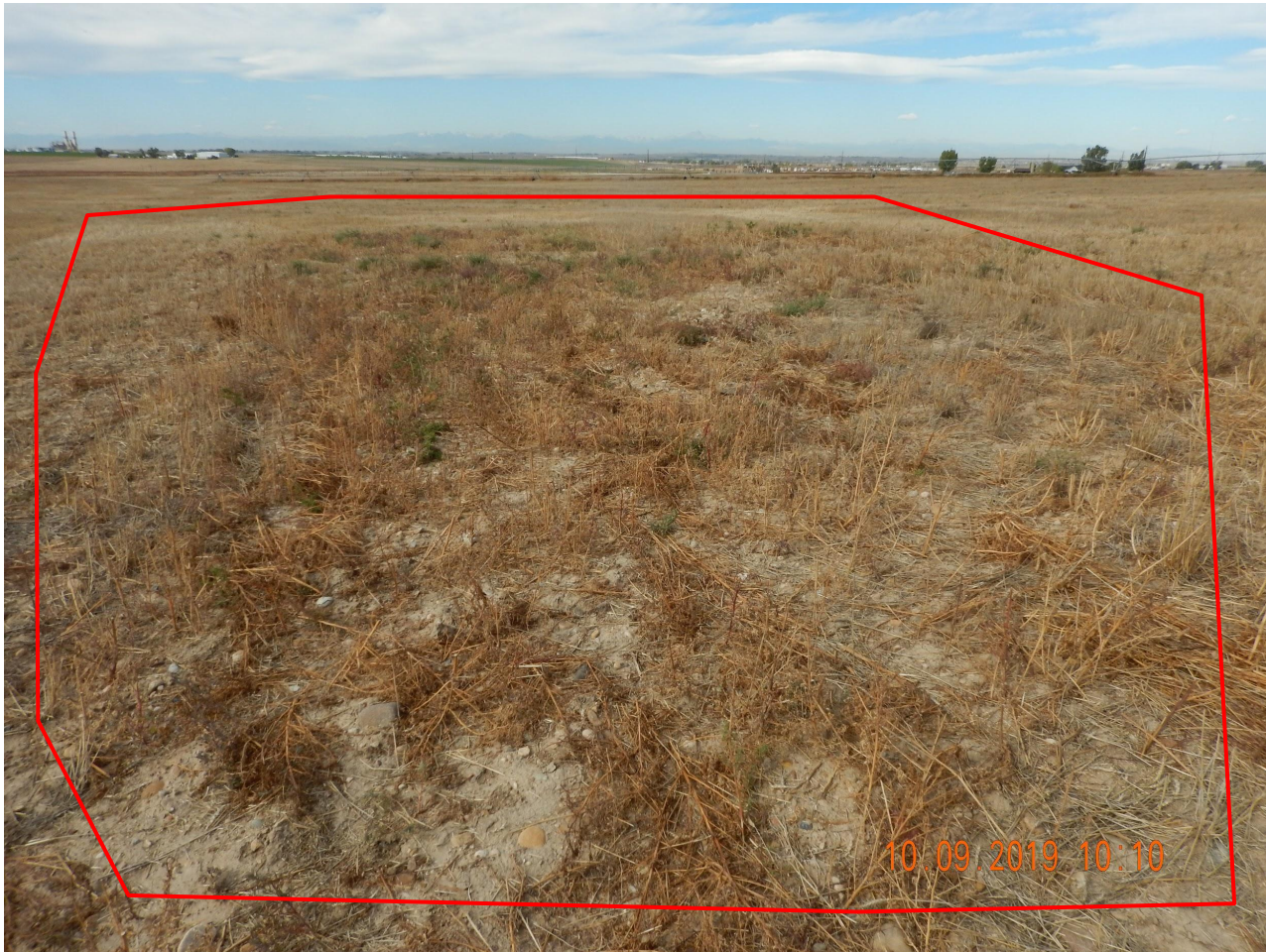
Photo 5. Photo taken from the well location, facing West. Photo illustrates the well location has not been properly recontoured and gravel was observed throughout portions of the disturbance area.
