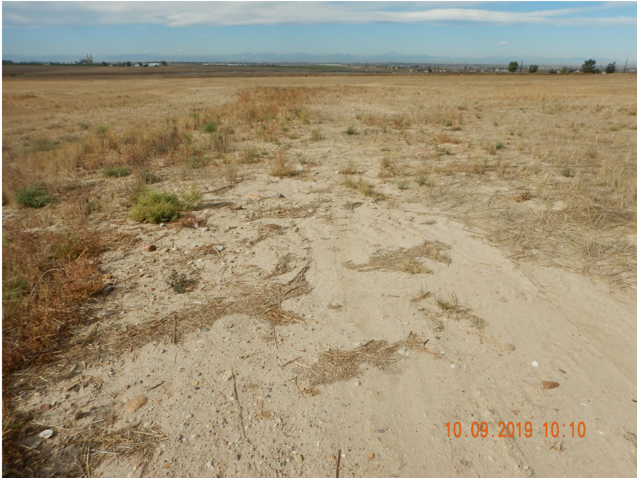
Photo 3. Photo taken from the southern well location access road, facing West. Operator has failed to properly recontour and reclaim the well location road.
