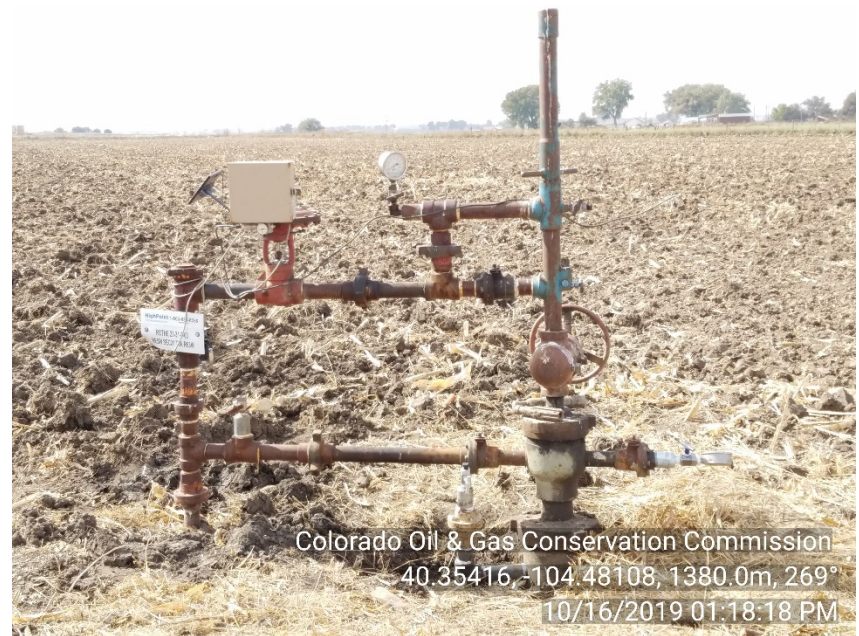
Photo #2 Rothe 23-31 Wellsite Temporarily Abandoned | TA Weeds NOW appear mitigated
