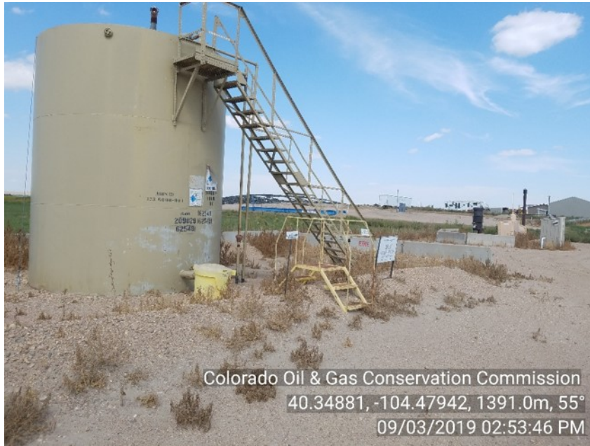
Photo #5 Rothe 24-31, 23-31 Battery Shut-down | Inactive Weeds prior insp.
