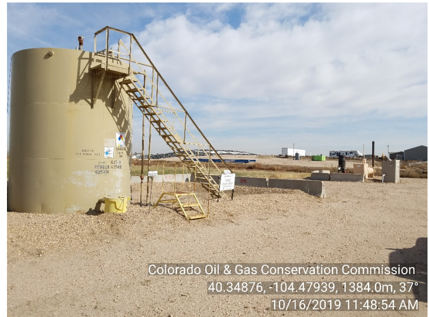
Photo #6 Rothe 24-31, 23-31 Battery Shut-down | Inactive Weeds NOW appear mitigated
