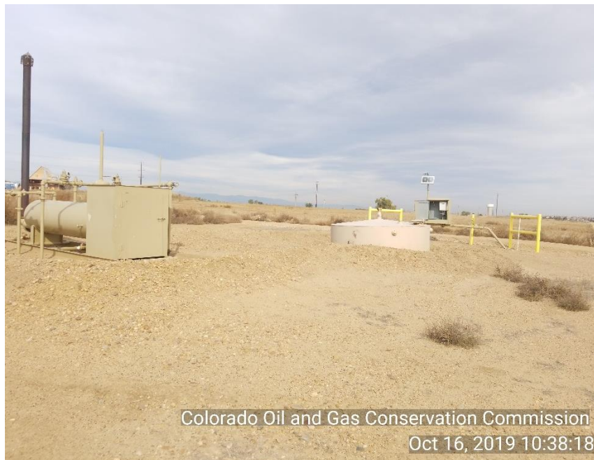
Photo 3 sep/ meter run and produced water tank
