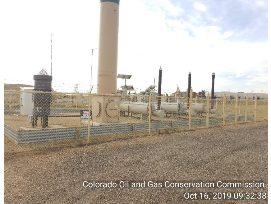
Photo 4 Sep/meter house and ECD's
