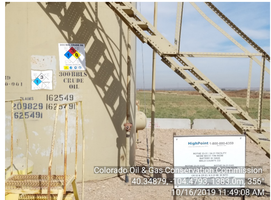
Photo #6 Rothe 24-31, 23-31 Battery Shut-down | Inactive NFPA label NOW legible
