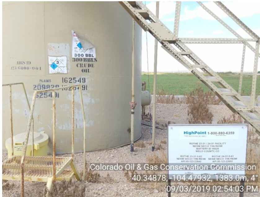
Photo #5 Rothe 24-31, 23-31 Battery Shut-down | Inactive NFPA Label peeling, NOT legible prior insp.
