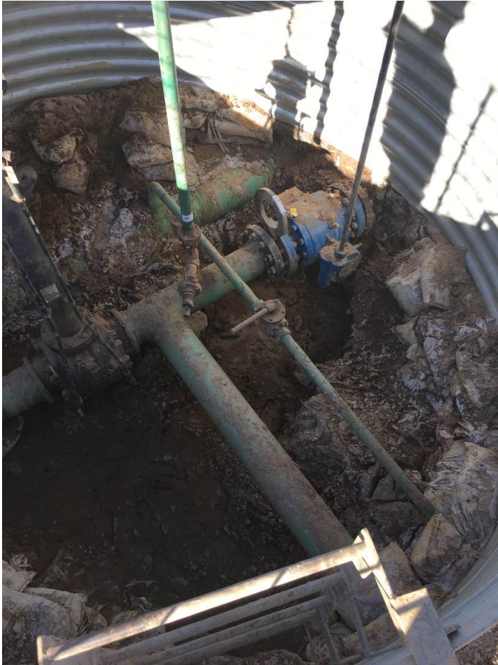
Release point at blue valve, Blank flange installed in picture with open flange on top
