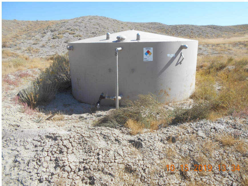
Tank with 2" riser inlet. Outlet disconnected and plugged.
