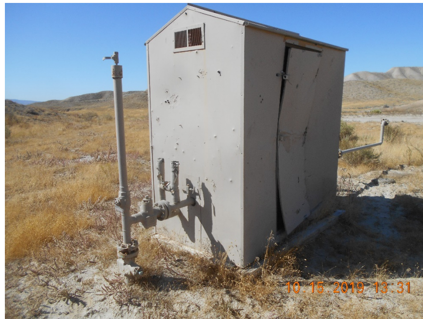
Valve locked with hammer union bull plug.
