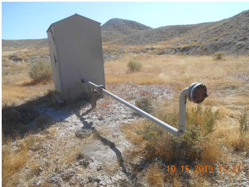
Meter housing with 2" blind flange.
