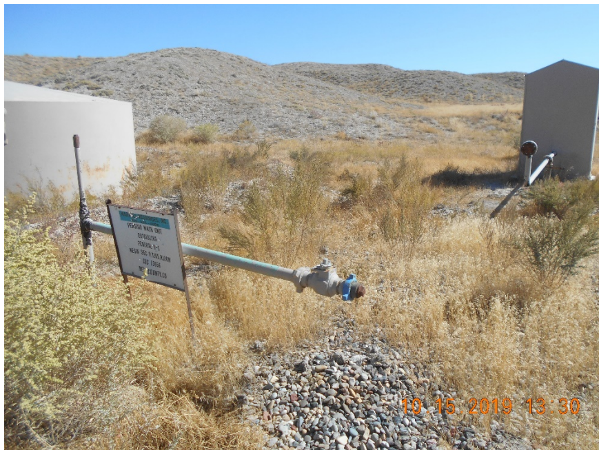
Sign with 2" riser. Valve locked with hammer union bull plug.
