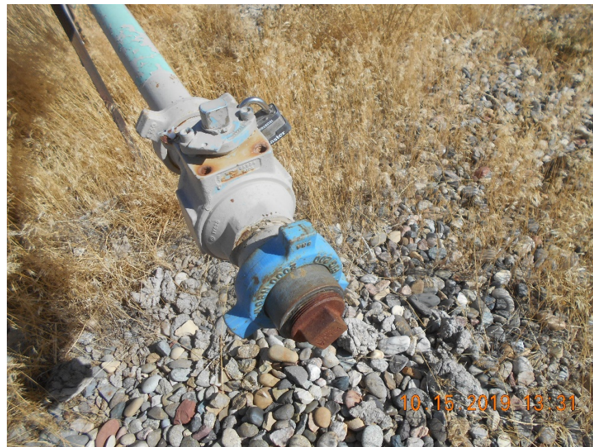
Valve locked with hammer union bull plug.
