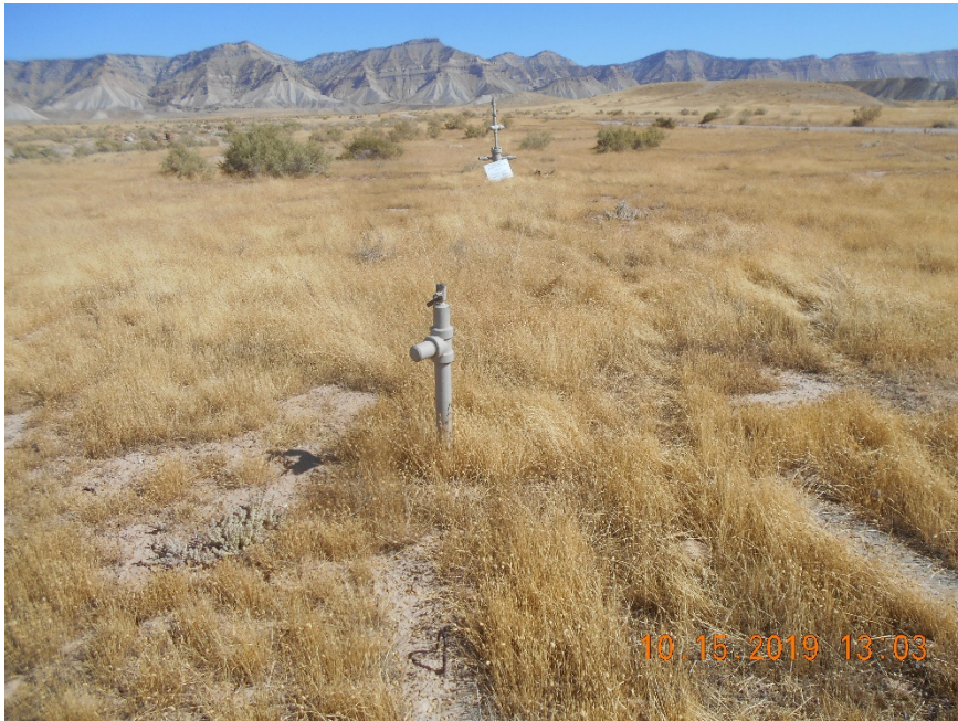
2" riser with bull plug and needle valve
