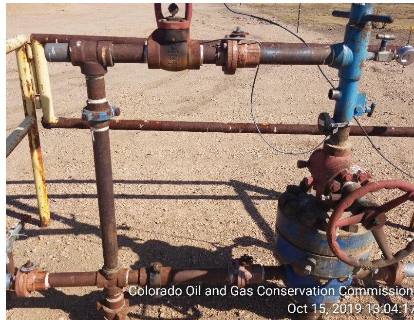
Photo 6 flow line valves are closed off well head
