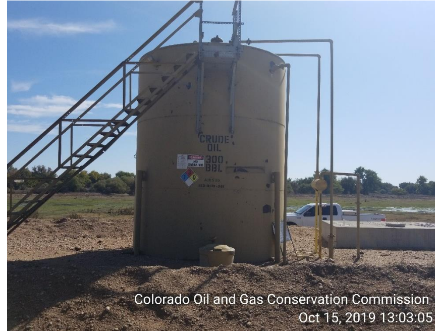
Photo 2 TNK BTRY 300 BBL crude oil tank does not have floodplain anchors. Produced water tank does have anchors.
