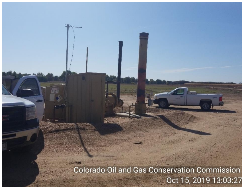
Photo 5 Sep/meter house and ECD. HOZ Sep has floodplain anchors
