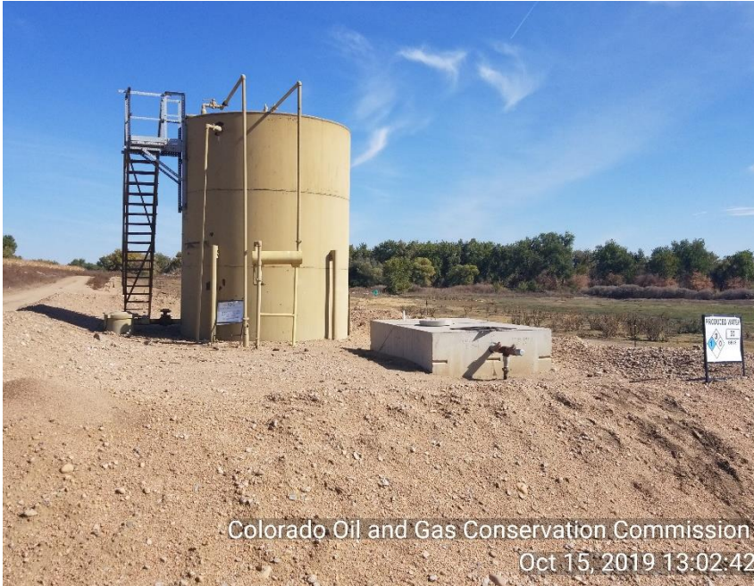
Photo 1 TNK BTRY 300 BBL crude oil tank does not have floodplain anchors. Produced water tank does have anchors.
