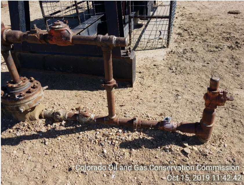
Photo 3 Flow line valves off well head are closed at time of inspection.
