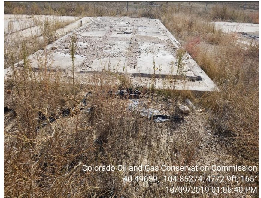
Photo 4 – Concrete slabs, trash and weeds
