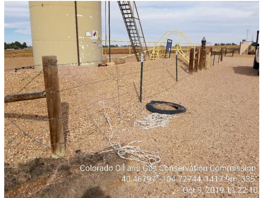
Photo 6: Debris (east of tank battery)
