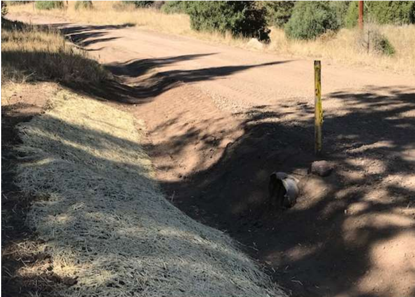
Photo 1: There was no erosion found up gradient of the culvert inlet. It appears that the established vegetation up gradient of the bar ditch was disturbed during the previous maintenance efforts. The sediment in the bar ditch is believed to have come from the earth disturbance. To correct this, the accumulated sediment was removed from the bar ditch. The disturbed soil was hand broadcast with an approved CPW seed mix to promote the establishment of vegetation. Erosion control blankets were installed for sediment control.
