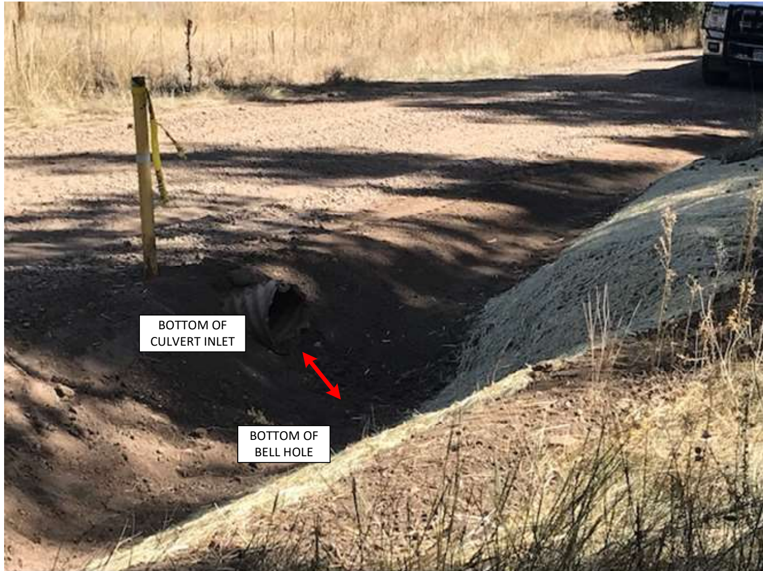
Photo 2: A bell hole was created below the culvert inlet to allow sediment time to drop out before entering the culvert inlet.
