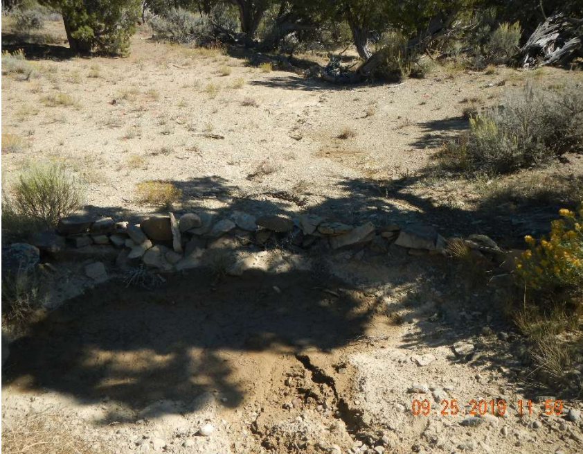
Photo #5 - View of the sediment catch located on the east side of the road.
