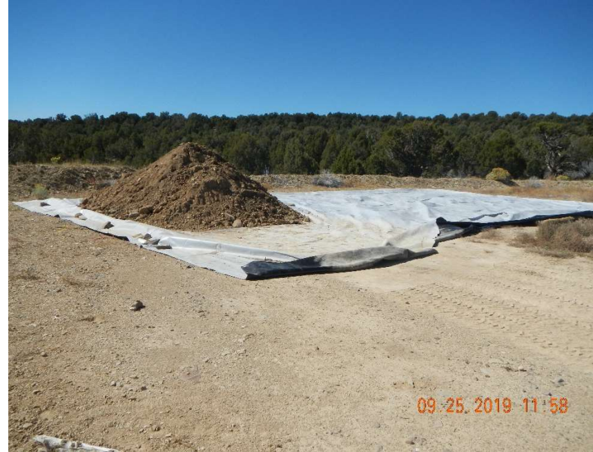
Photo #8 – View of the contaminated stock piled soil.
