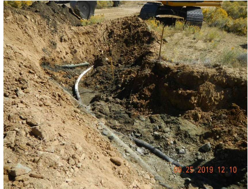
Photo #2 – View of the excavation with the 4-inch (produced water) and 6-inch flowlines (gas).
