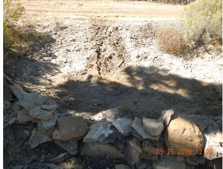
Photo #4 – View of the sediment catch located on the east side of the road.
