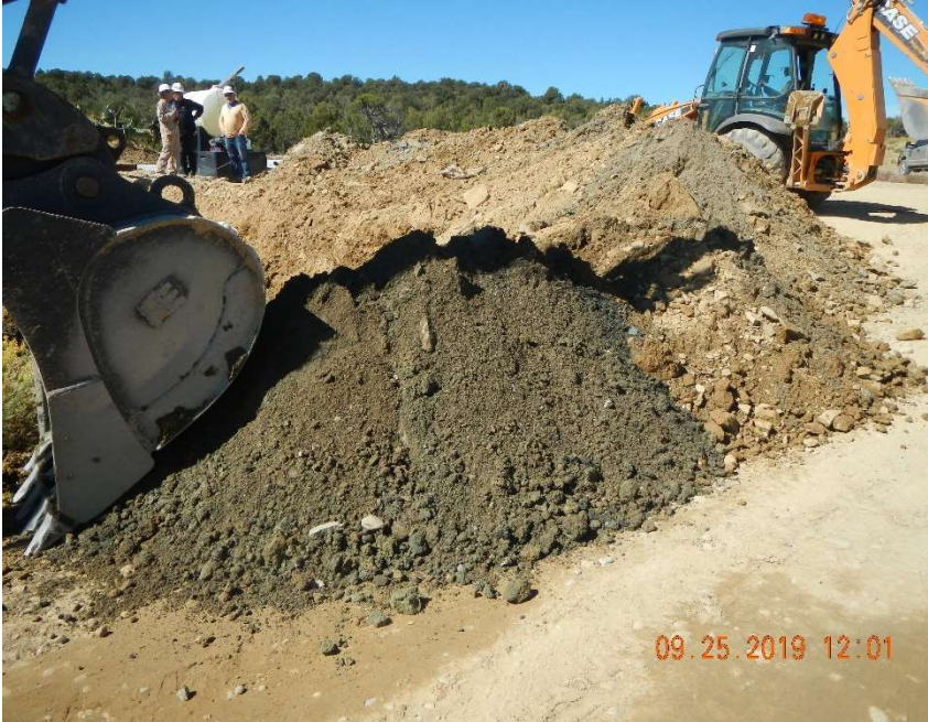
Photo #7 – View of the flowline bedding that was excavated.
