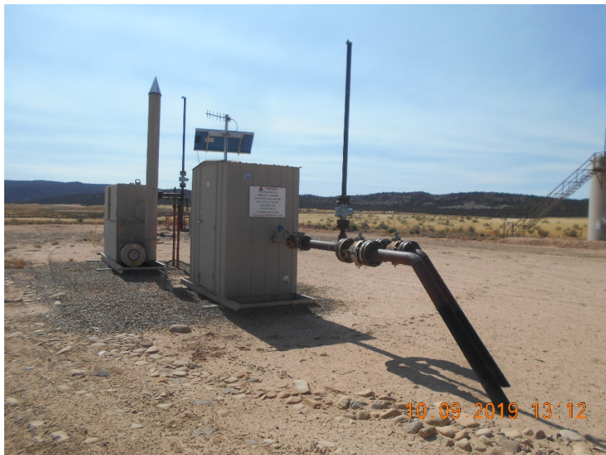
Meter housing with sign and Separator
