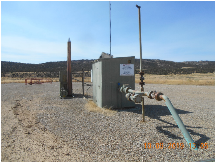
Meter housing with sign and Separator
