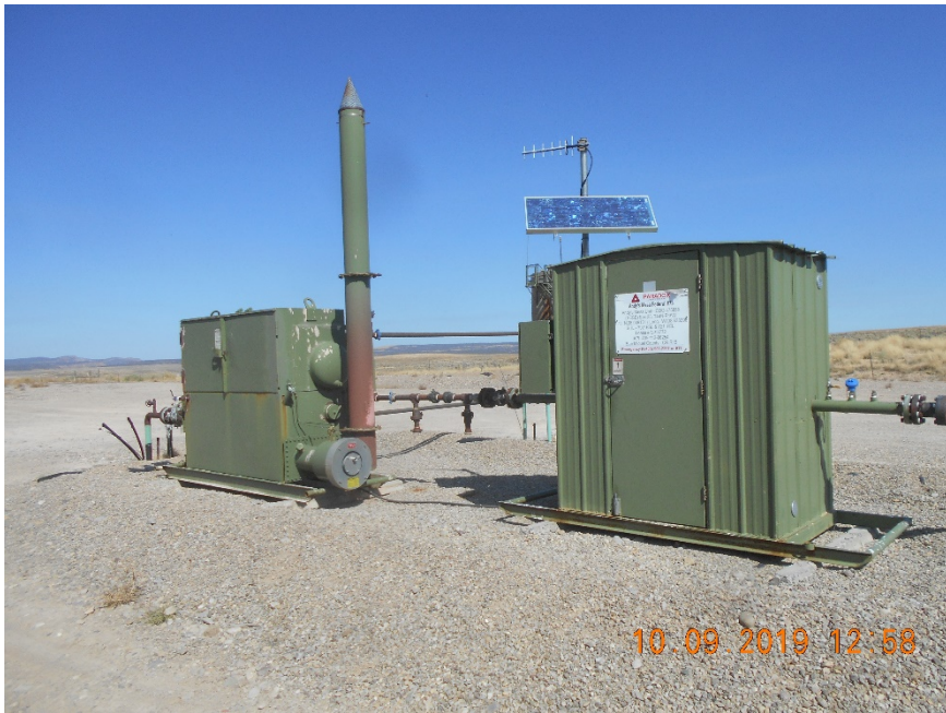
Meter housing with sign and Separator
