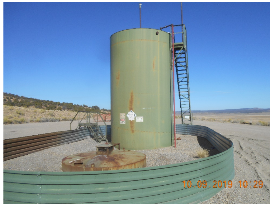
Produced water and Condensate tank battery
