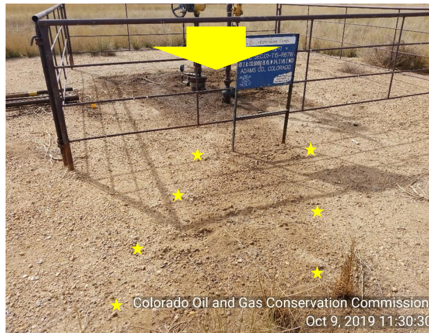
Photo 2 Stained soil around well head and on site
