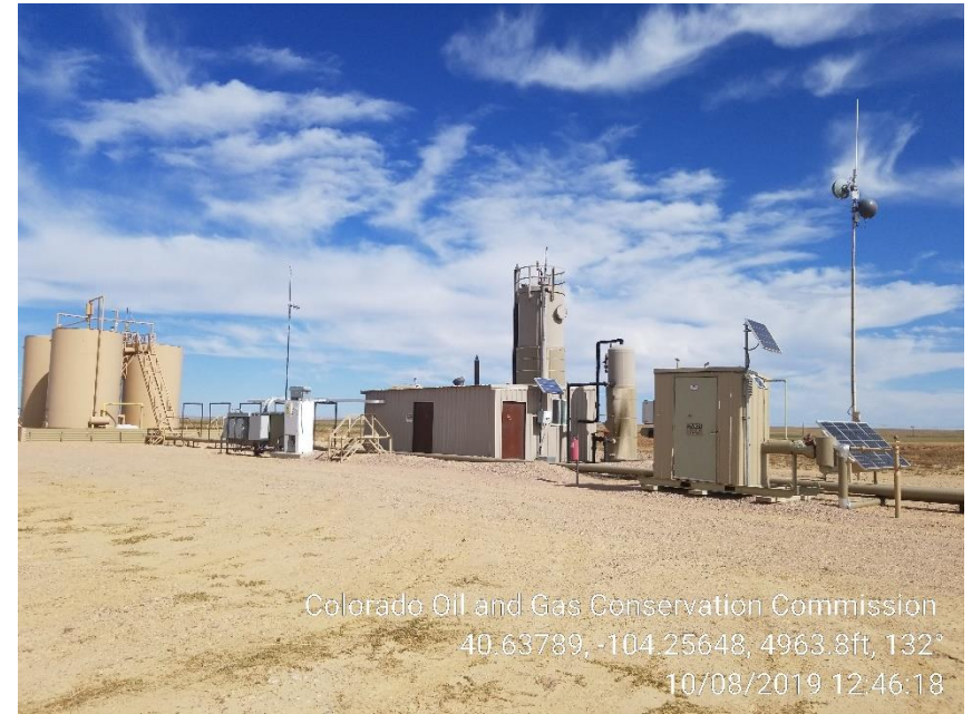
Photo 2 – Tank Battery
