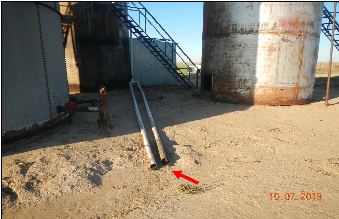
Photo 4. These pipe have oily waste at the ends with no containment. The tank on the right is not in use and is considered unused equipment.
