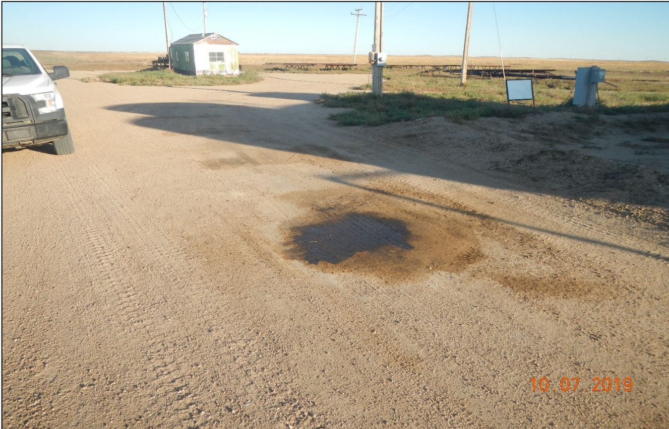
Photo 2. There is oil stained soil on the road surface near the tank battery. Approximately 4 ft. x 4 ft. area.
