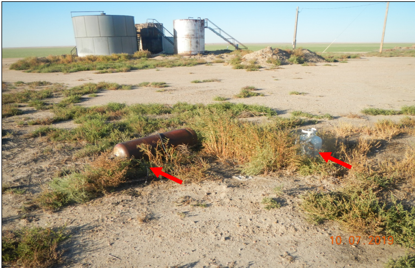
Photo 5. There are propane tanks at the south side of the location which is a safety concern and are not properly stored.
