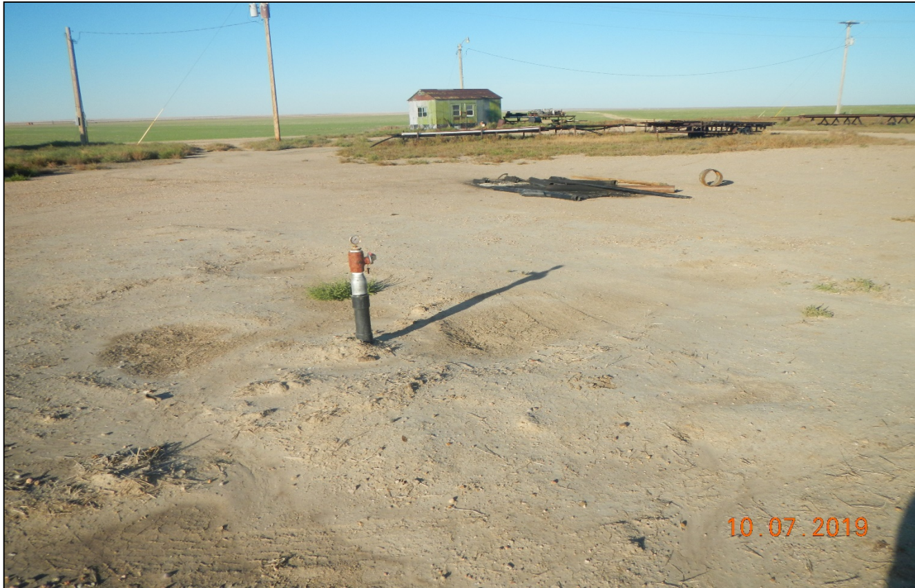
Photo 7. Facing northeast at the south side of the location. Pipe risers at the south side of the location have no LO/TO and are not protected from vehicle striking hazard.
