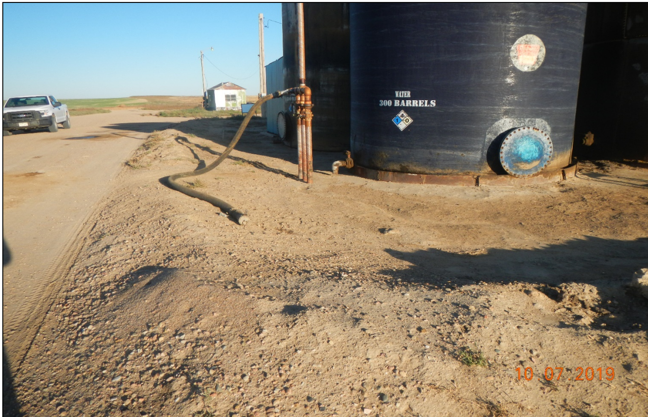
Photo 3. The berms around the tanks are worn down and not adequate to contain a spill.
