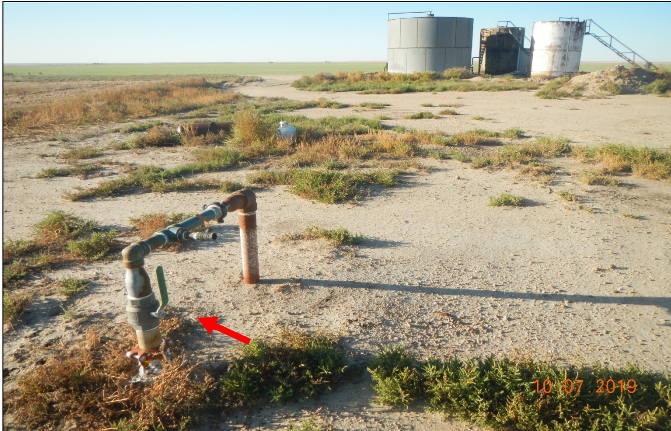
Photo 6. Pipe risers at the south side of the location have no LO/TO and are not protected from vehicle striking hazard.
