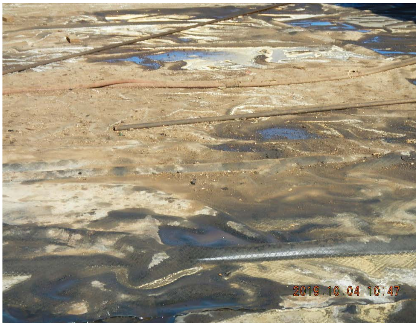
Oily water/fluids pooled on liner in secondary containment, 1" by app 30' pipe directly on liner of secondary containment.
