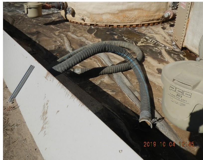
Delivery hose directly on liner of secondary containment.
