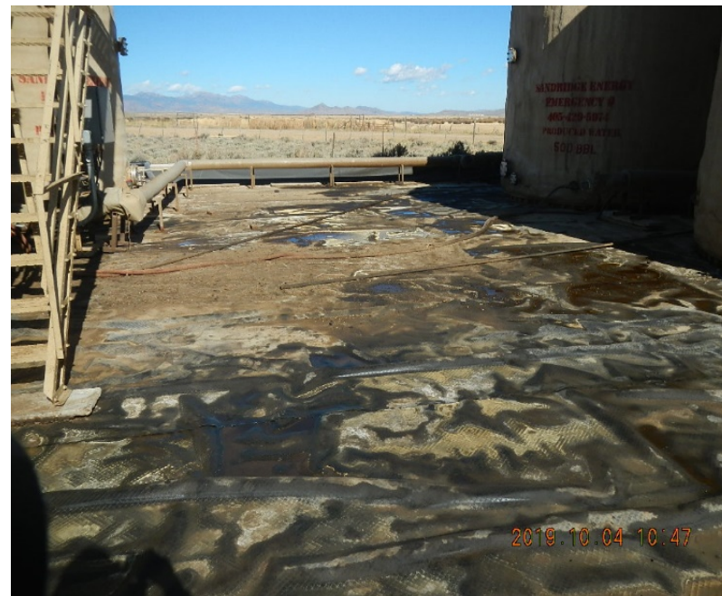
Oily water/fluids pooled on liner in secondary containment, 1" by app 30' pipe directly on liner of secondary containment.
