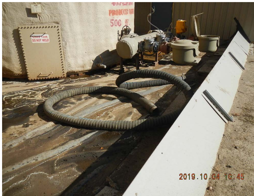
Delivery hose directly on liner of secondary containment and residual oil and salt staining.
