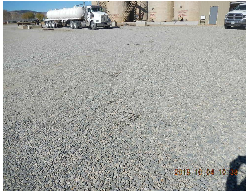
Stained soil/gravel in multiple areas of Location and vehicle tracking.
