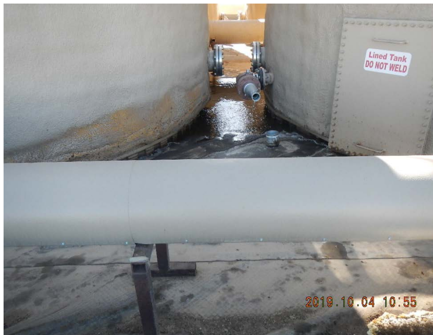
Oily water/fluids pooled on liner in secondary containment. Uncapped valve with bull plug on liner.
