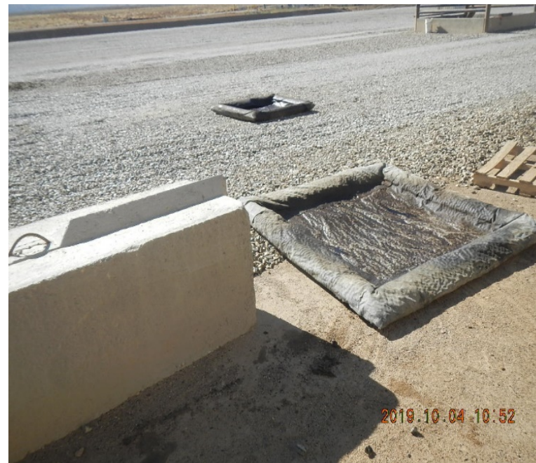
Drips and staining of oil on the recently placed gravel at the load out area and oily soaked catch mats.
