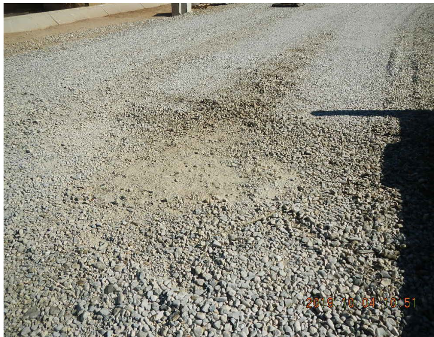
Drips and staining of oil on the recently placed gravel at the load out area.
