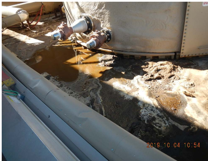
Oily water/fluids pooled on liner in secondary containment and sorbent material.
