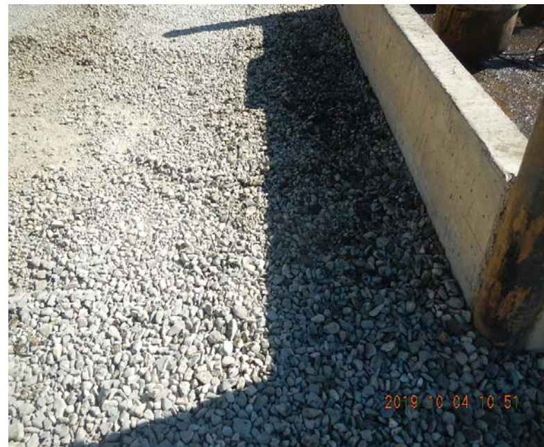
Drips and staining of oil on the recently placed gravel at the load out area.
