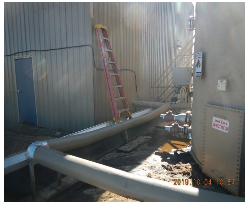
Oily water/fluids pooled on liner in secondary containment and sorbent material. Improper storage of ladder.
