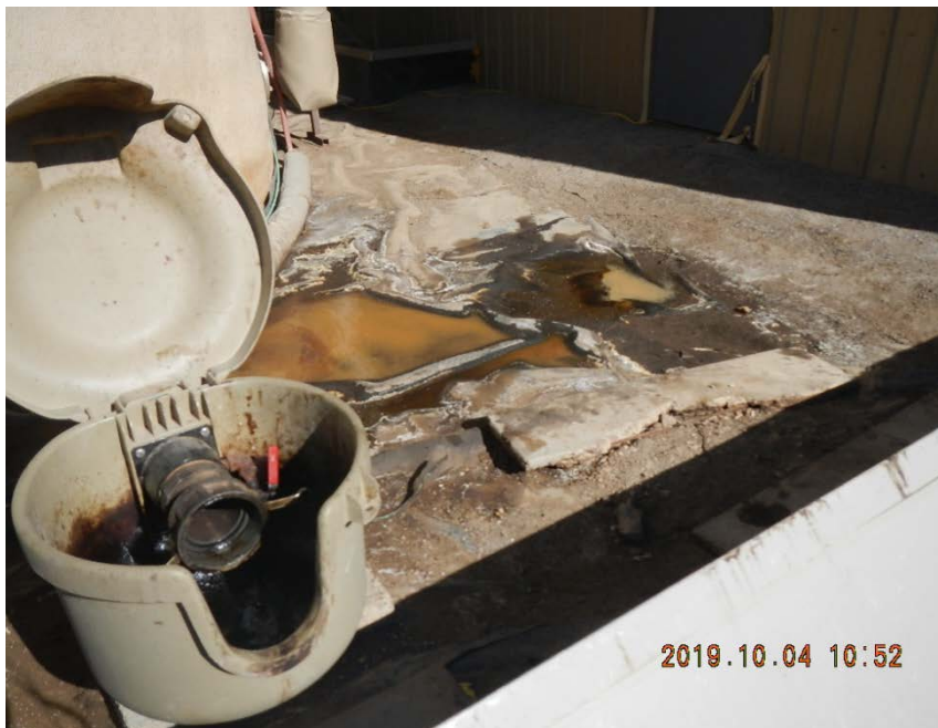
Oily water/fluids pooled on liner in secondary containment.
