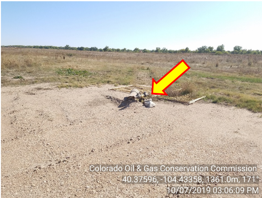
Photo #1 Huck 41-28 (05-123-21882) Wellsite Plugged & Abandoned | PA Appears to be cut & capped Unused Equipment Unused flow line riser NOT marked & LO/TO
