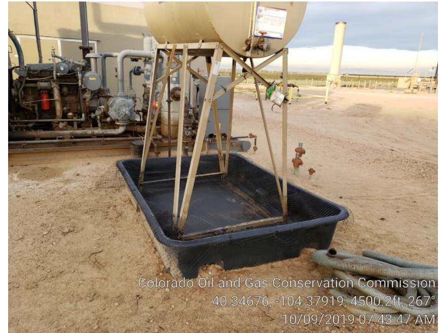
Photo # Oily water in containment for Compressor oil tank. On 10/9/19
