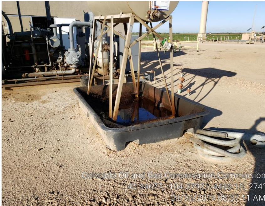
Photo # Oily water in containment for Compressor oil tank. On 9/30/19
