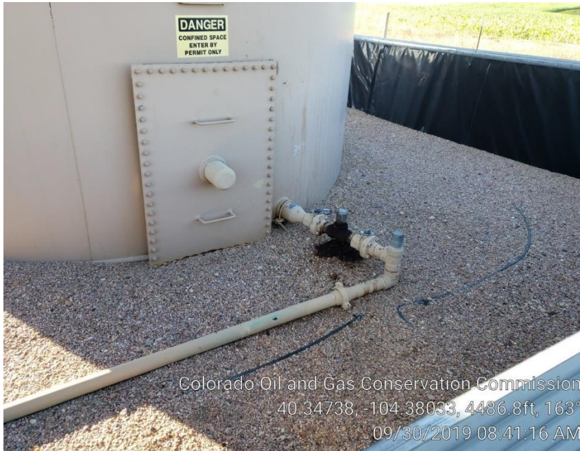
Photo # Oily waste. Stained soil appears at crude oil tanks in multiple areas. On 9/30/19
