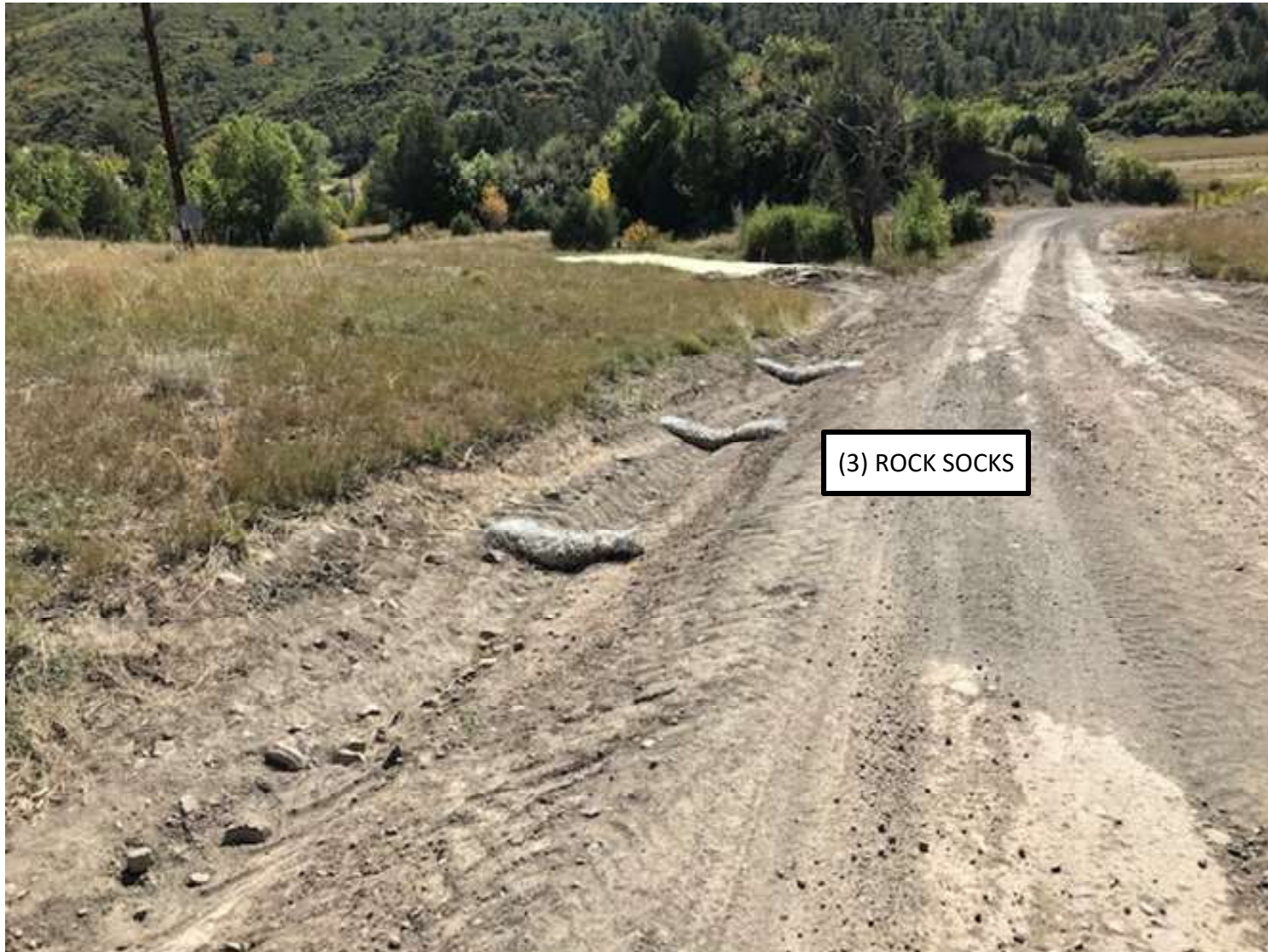
Photo 5: (3) Rock socks were placed in the bar ditch to filter out sediment during periods of run off.
