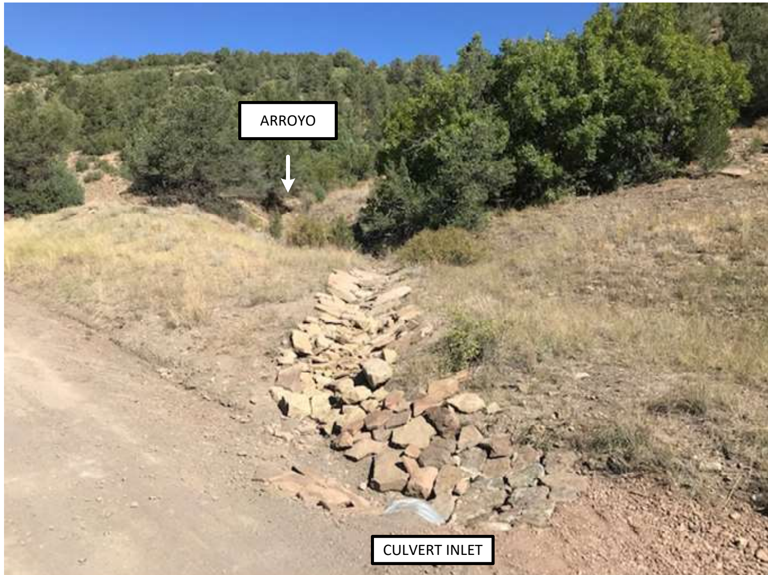
Photo 2: Culvert installed and the arroyo lined with rip rap to diffuse energy.
