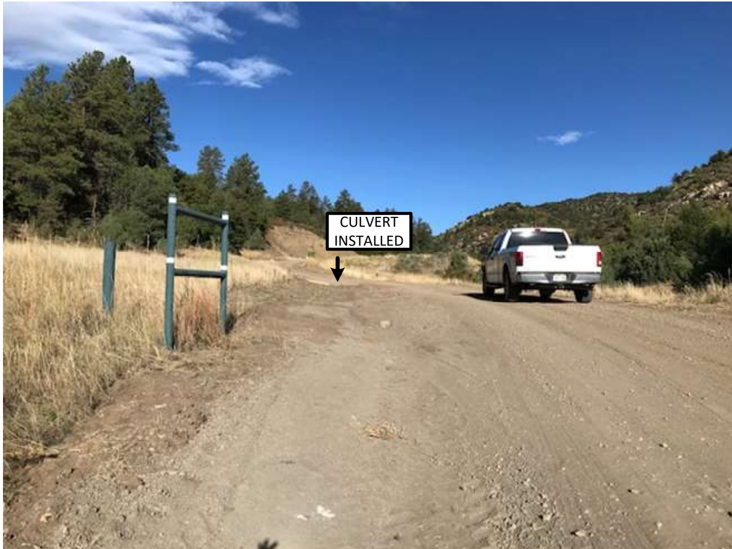
Photo 7: The rock check dams were removed from the bar ditch. The channelized area of the ditch was reshaped into a parabolic shape. A culvert was installed up gradient of this area to reduce the amount of run off the bar ditch would receive.
