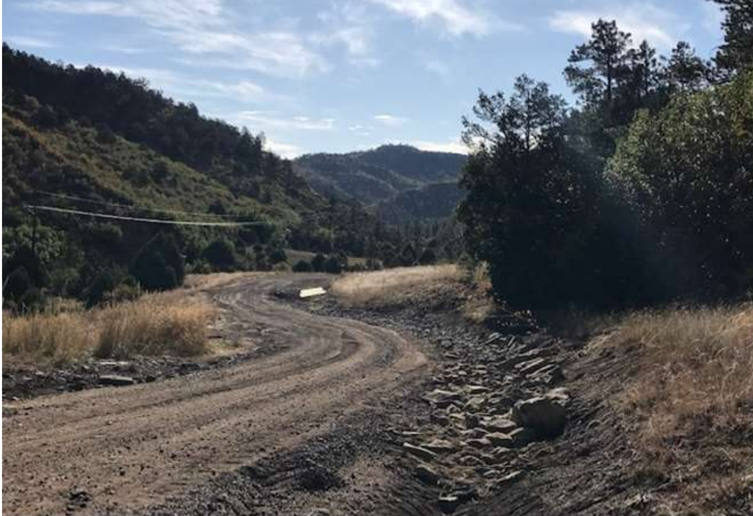
Photo 9: Rip rap was installed in the portion of the bar ditch that was steep to dissipate energy from run off.
