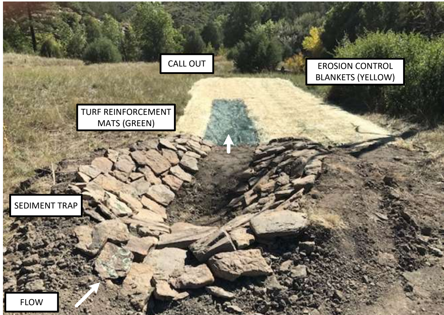
Photo 6: A sediment trap was installed at the end of the bar ditch where run off is directed to a call out. The sediment trap will allow time for the sediment to drop out from run off. Rock was installed to dissipate energy and stabilize the soil. Turf reinforcement mats were installed below the sediment trap where run off is concentrated to control erosion. Erosion control blankets were installed for soil stabilization, where run off would sheet flow. An approved CPW seed mix was hand broadcast to promote the establishment of vegetation.
