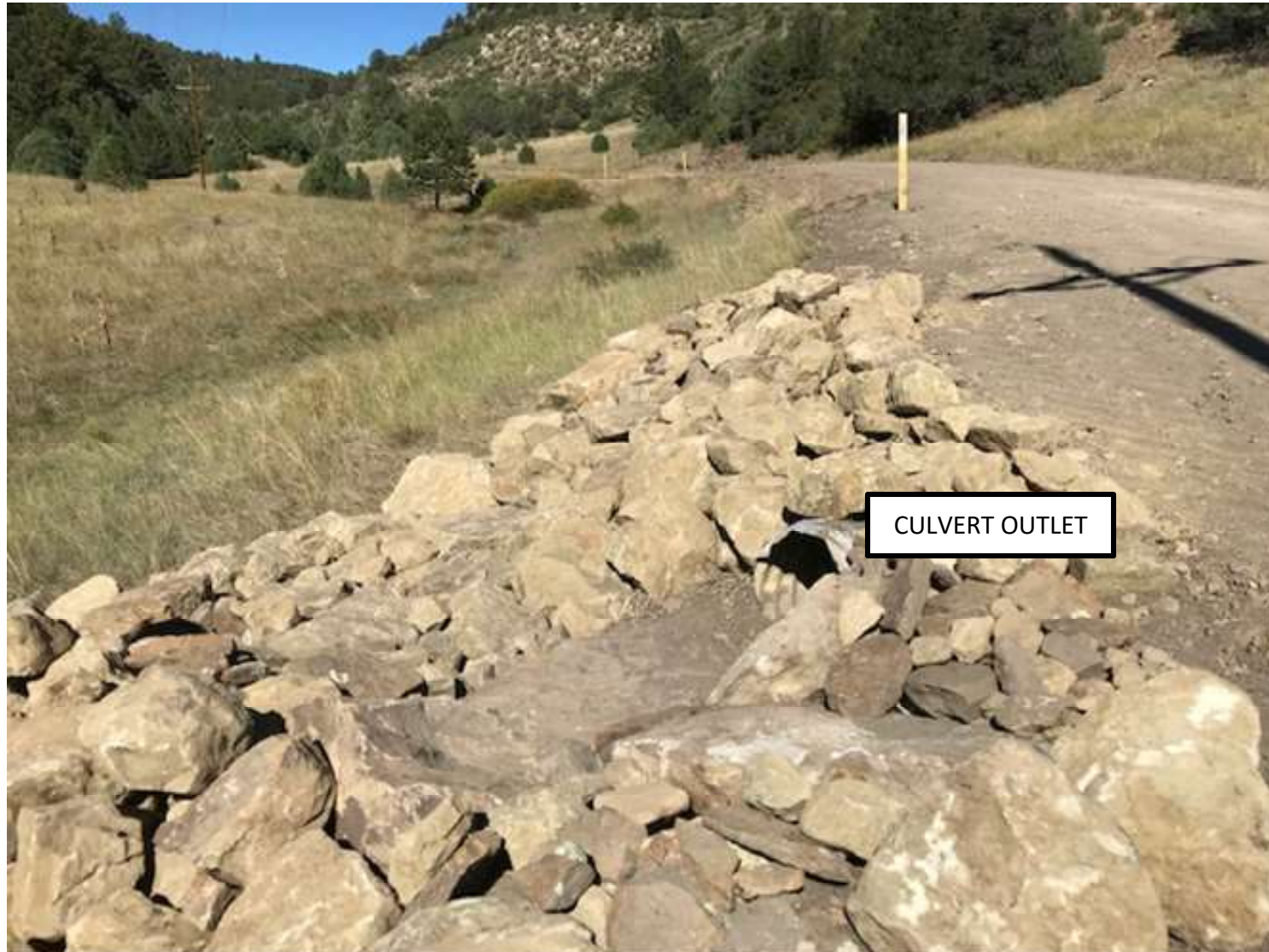
Photo 4: The culvert outlet was armored to prevent erosion from run off.
