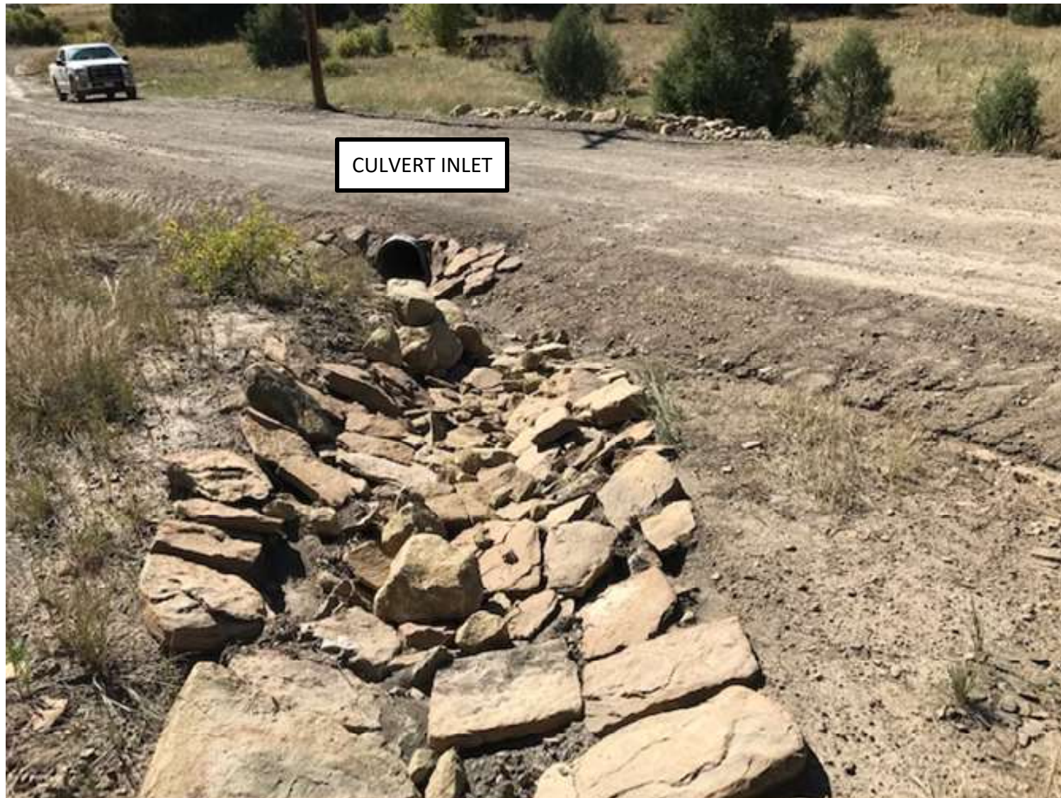
Photo 3: Culvert installed and the arroyo lined with rip rap.
