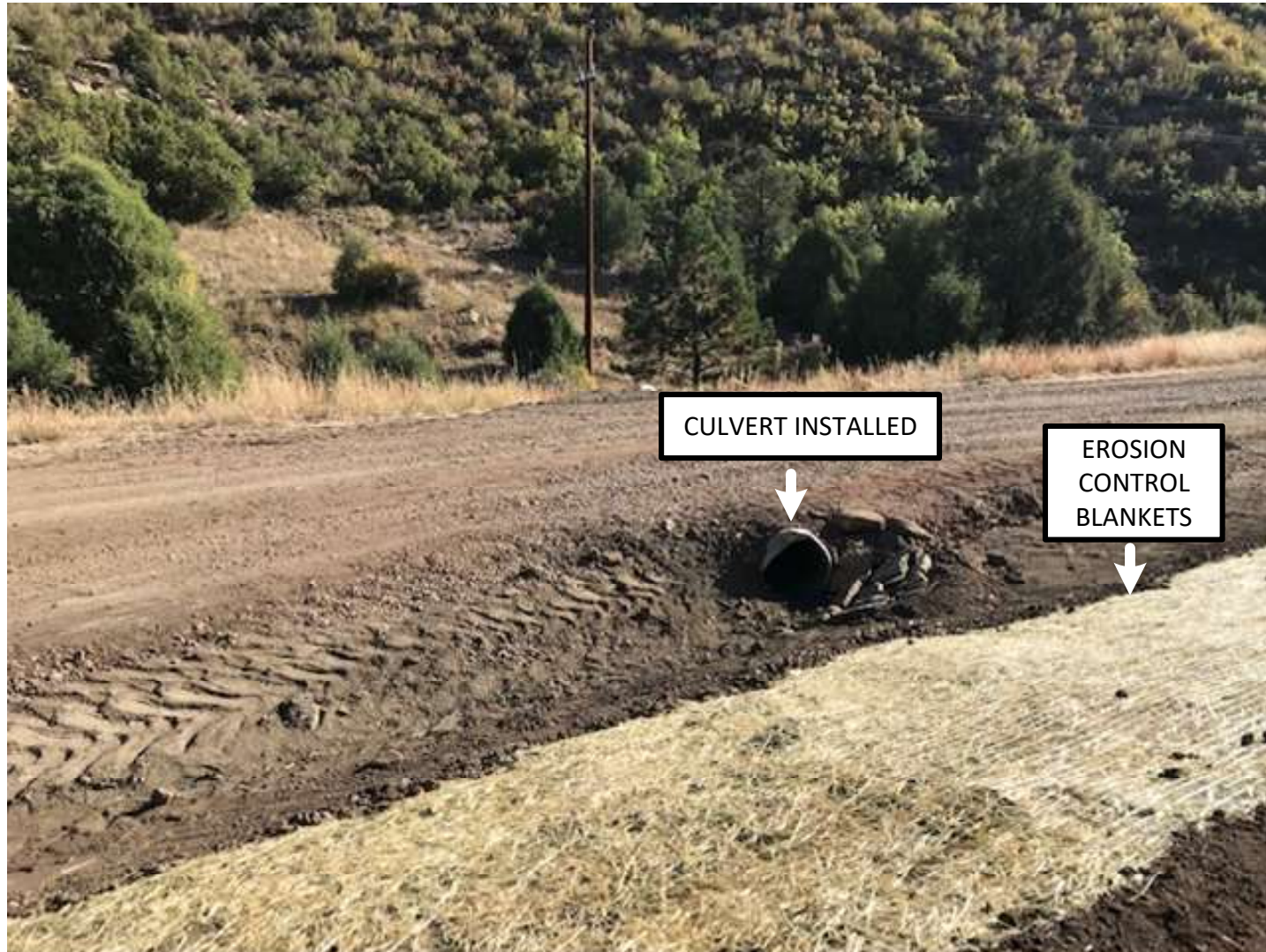
Photo 8: The rock check dams were removed from the bar ditch. The channelized area of the ditch was reshaped into a parabolic shape. A culvert was installed to reduce the amount of run off the bar ditch would receive down gradient of the culvert. Erosion control blankets were installed for soil stabilization where the earth was disturbed. An approved CPW seed mix was hand broadcast to promote the establishment of vegetation.
