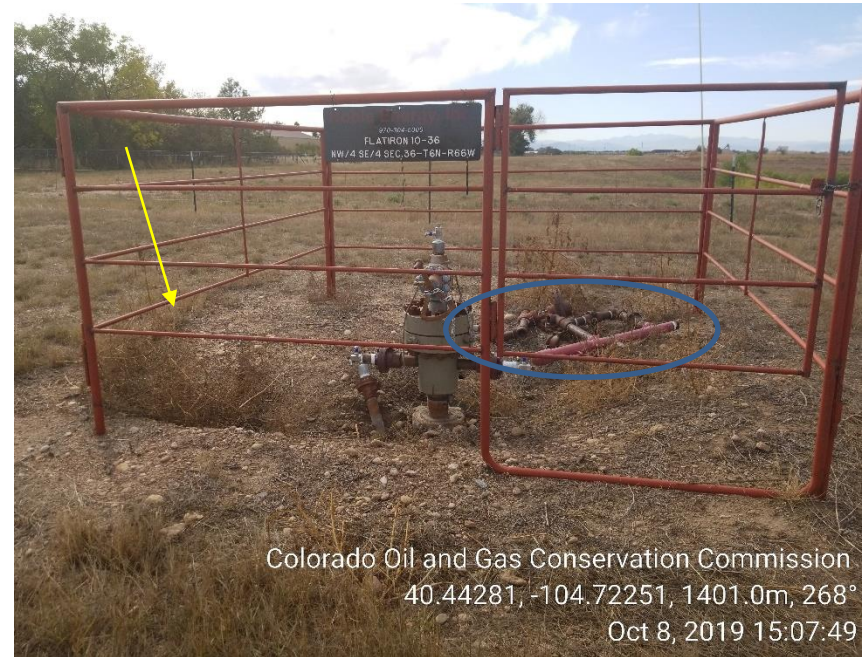
Photo 2: Wellhead; UNUSED EQUIPMENT; DEBRIS/WEEDS; NO ORANGE DECOMMISSION SIGN
