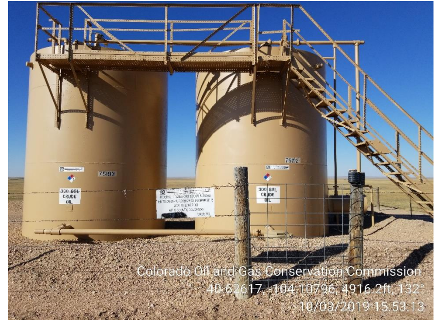
Photo 2 – Tank Battery – Tanks Repairs and Painted per Previous Inspection 691200732
