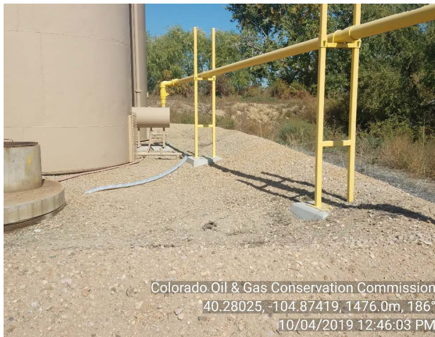
Tank berm on 10/4/19
