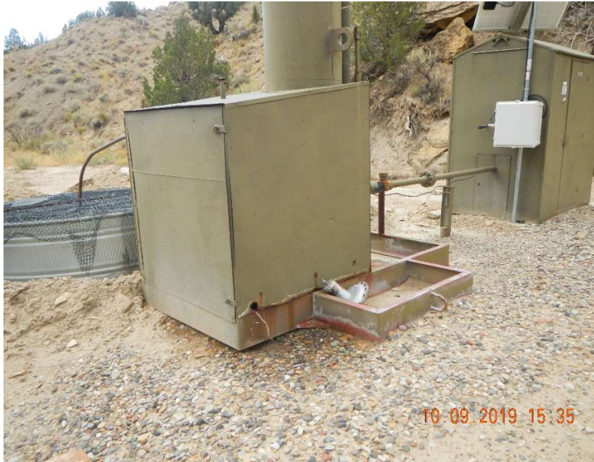
Photo #5 – Stained soil beneath vertical separator.
