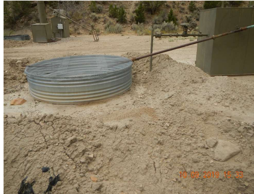
Photo # - Unlabeled stock tank east of horizontal separator.
