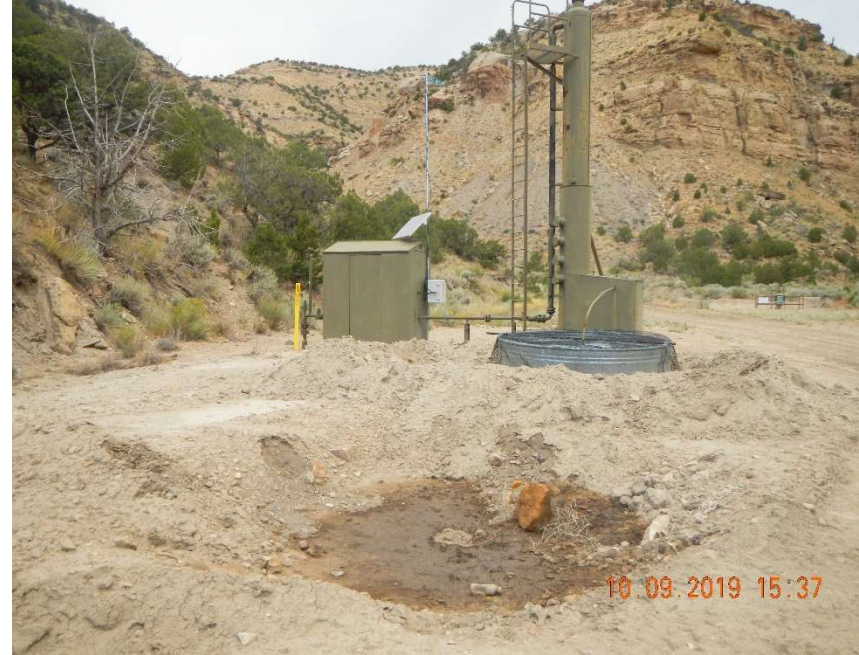
Photo #8 – View of the pit 10 feet by 10 feet by 3 feet deep pit located east of the vertical separator.
