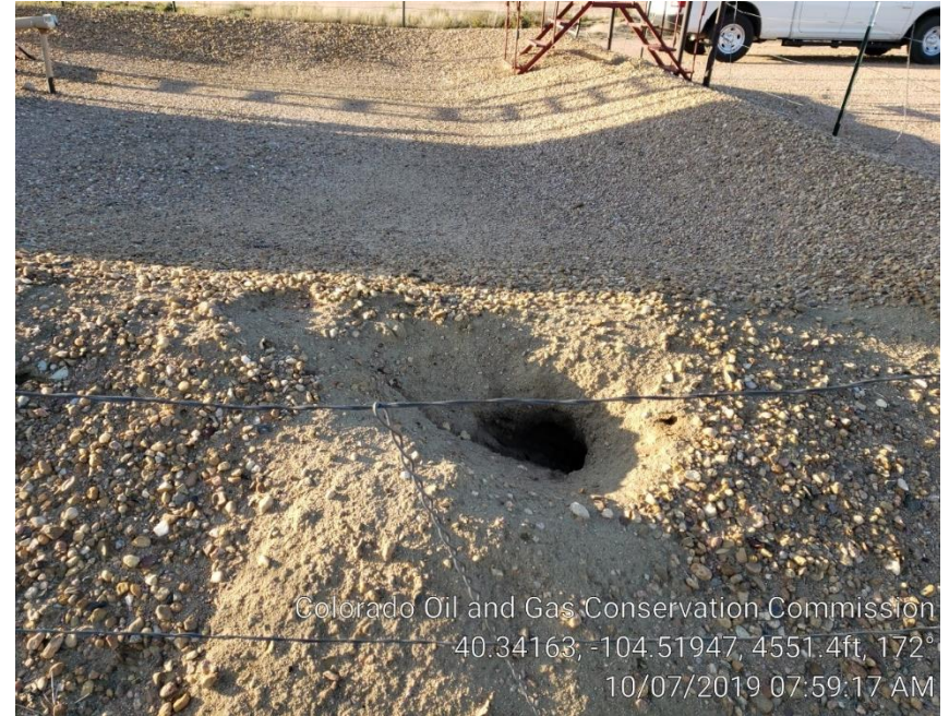
Photo #6 Animal hole in berm
