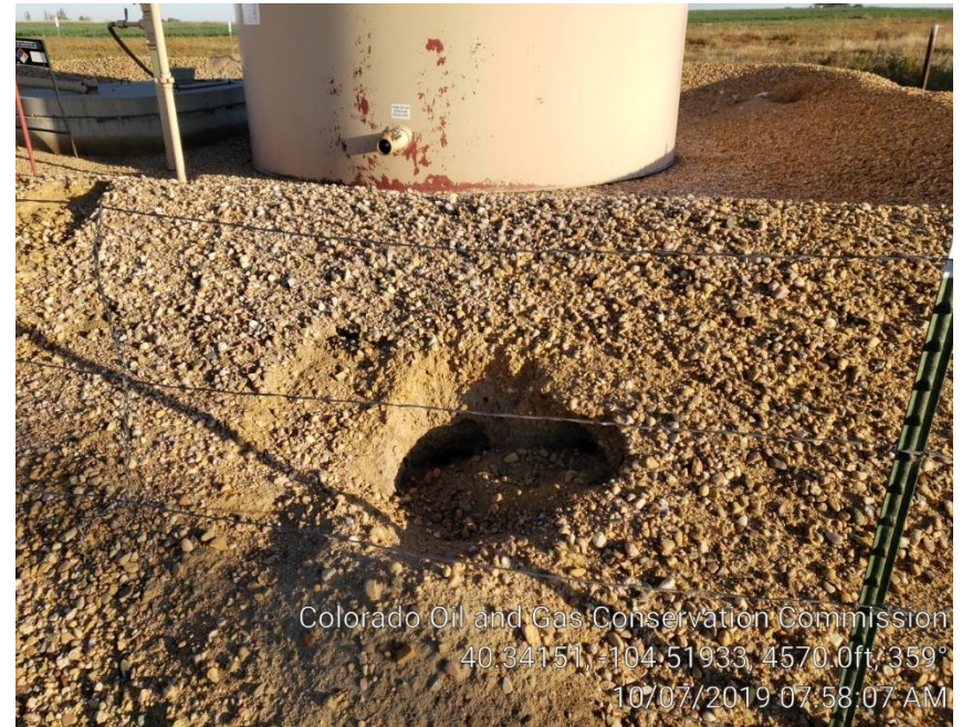
Photo #4 Animal hole in berm
