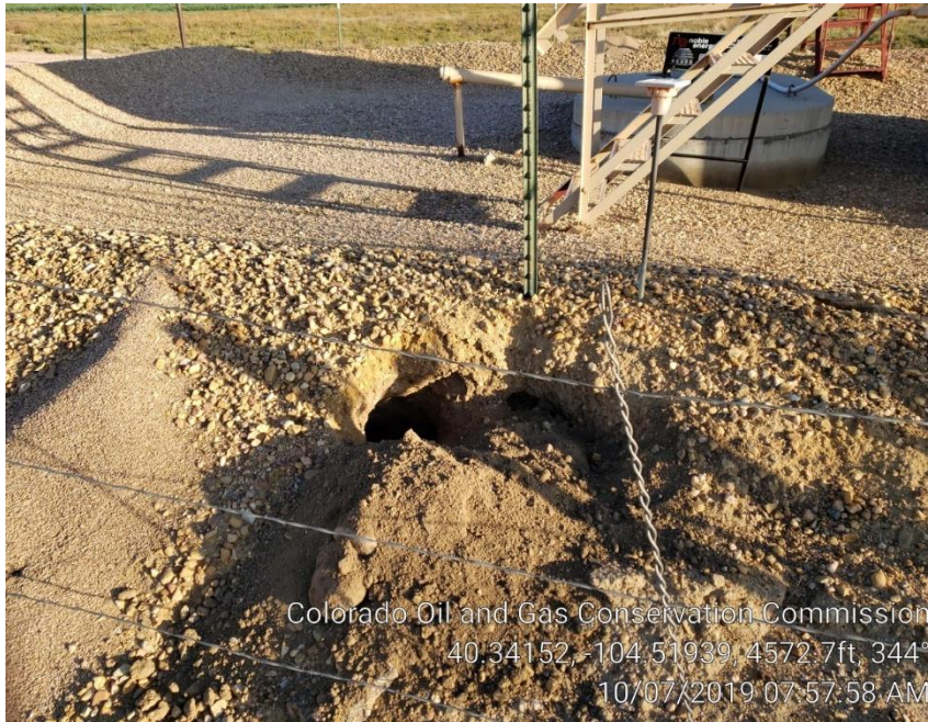
Photo #3 Animal hole in berm
