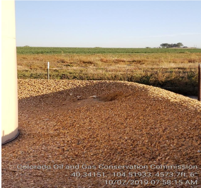
Photo #5 Animal hole in berm
