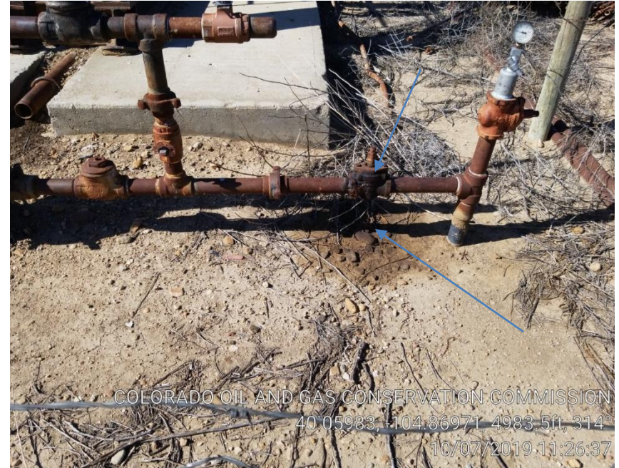
Pic 2 stained soil/mechanical issue
