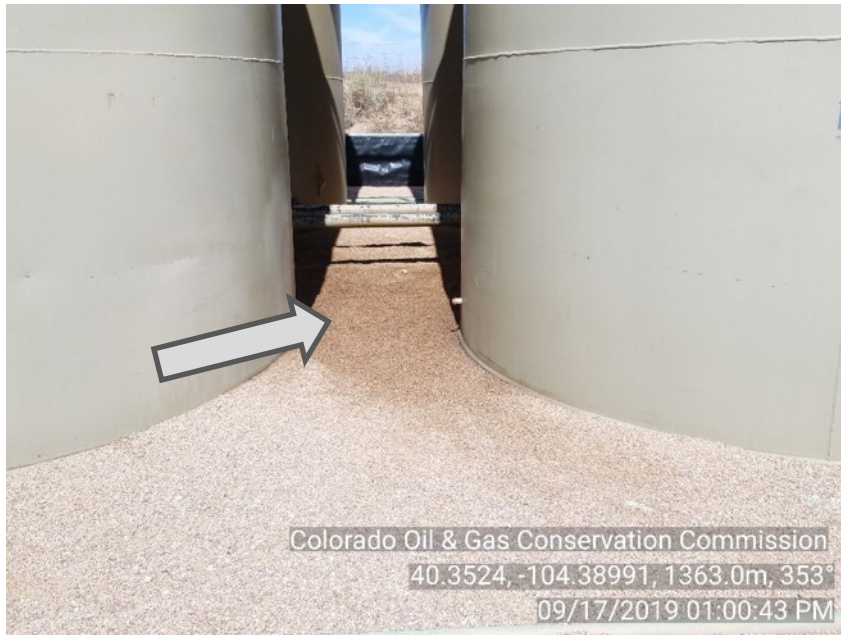
Photo #6 North Platte 14-36, X-D-35HZ Battery Latham F-J-35HZ Crude oil tanks 2, 3 Stained soil prior insp.
