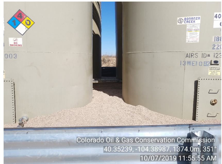
Photo #7 North Platte 14-36, X-D-35HZ Battery Latham F-J-35HZ Crude oil tanks 2, 3 Stained soil NOW appears mitigated
