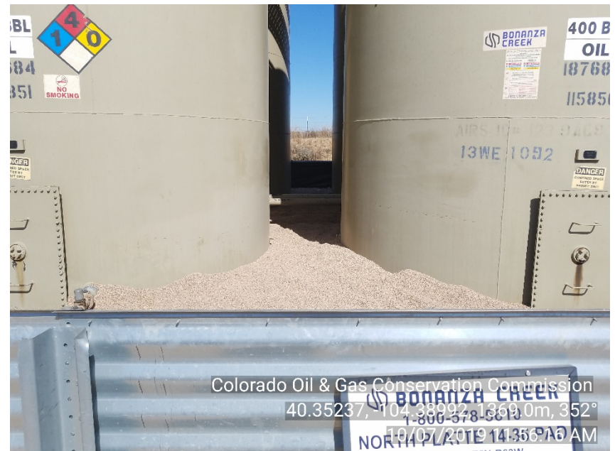
Photo #9 North Platte 14-36, X-D-35HZ Battery Latham F-J-35HZ Crude oil tanks 3, 4 Stained soil NOW appears mitigated
