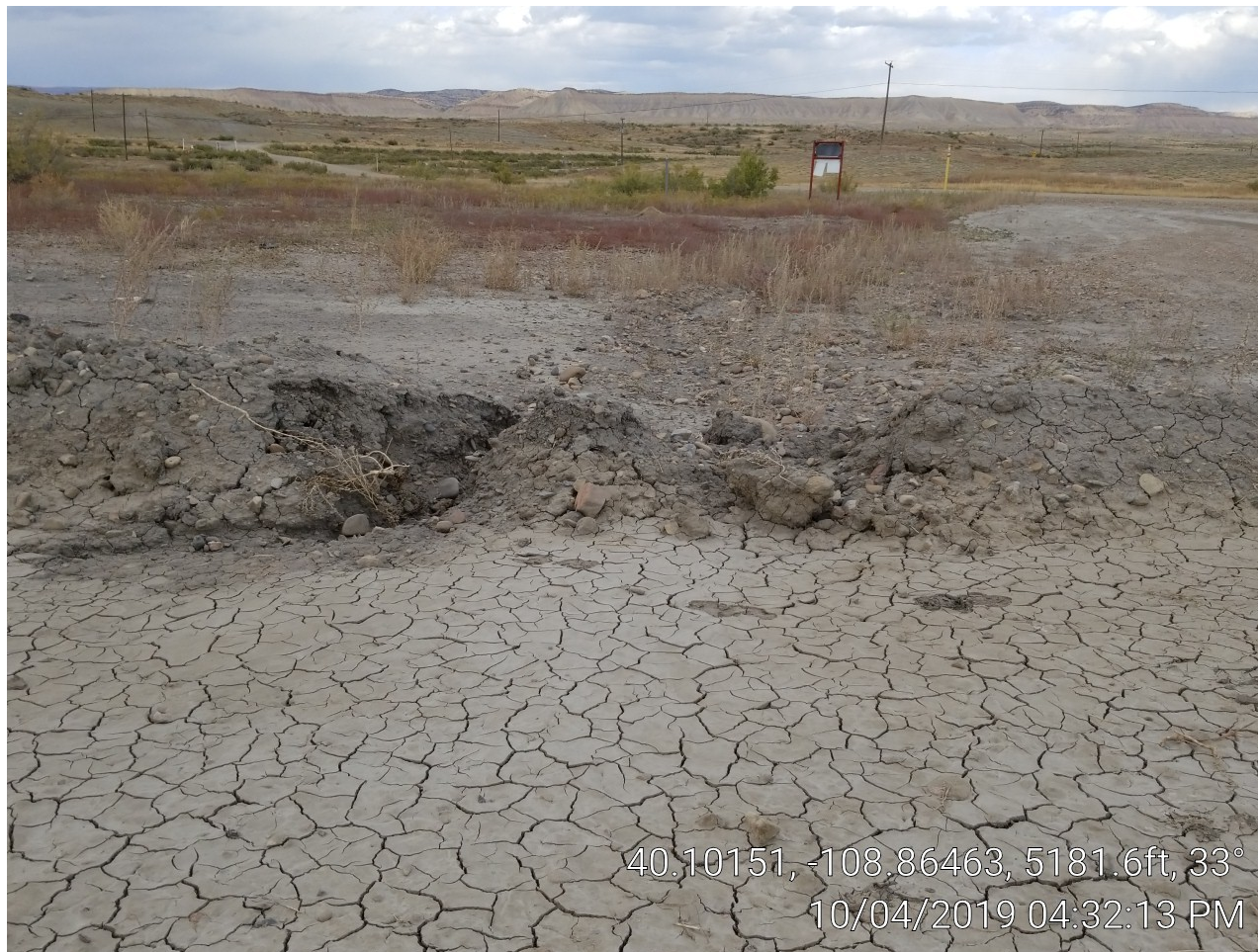
Photo 2. Break in location berm.
