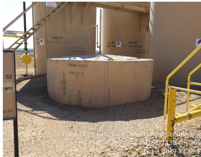
Photo 14: No NFPA placard on produced water tank
