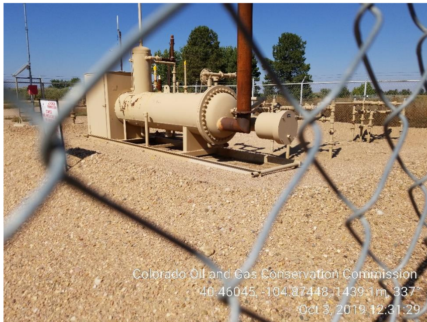
Photo 13: Separator NOT anchored
