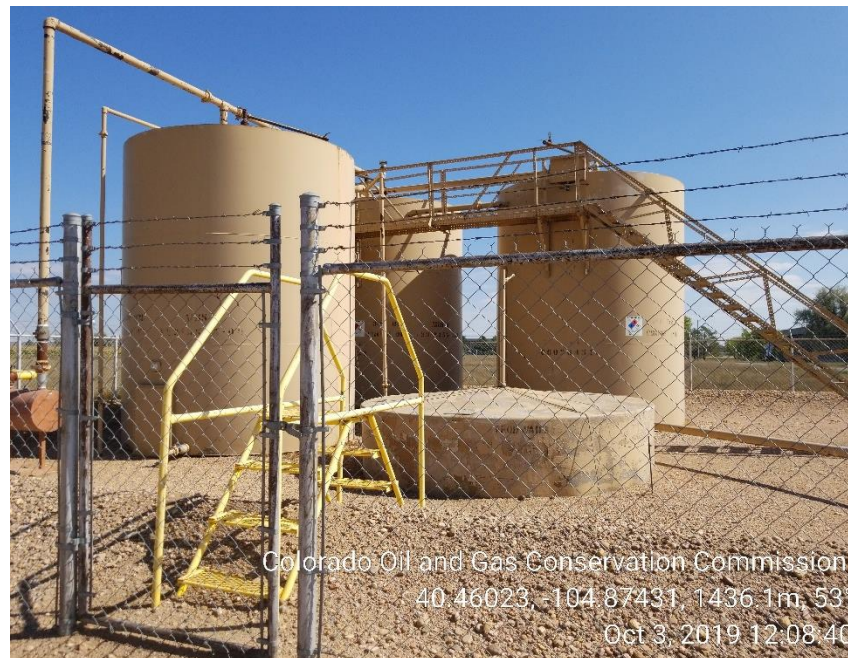
Photo 12: Tanks NOT anchored
