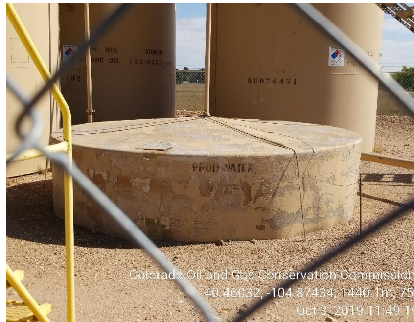
Photo 14: No NFPA placard, BBLS faded on H2O tank
