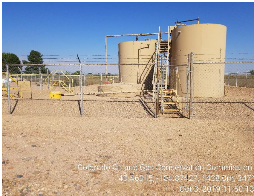
Photo 11: Tank Battery, Inadequate containment surrounding tank battery
