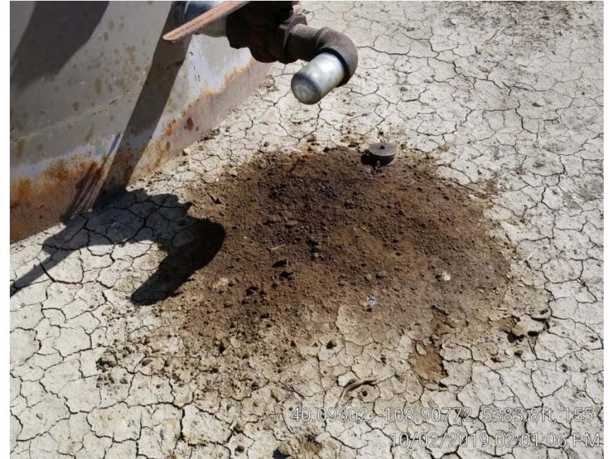
Photo 3. Stained soil next to tank.
