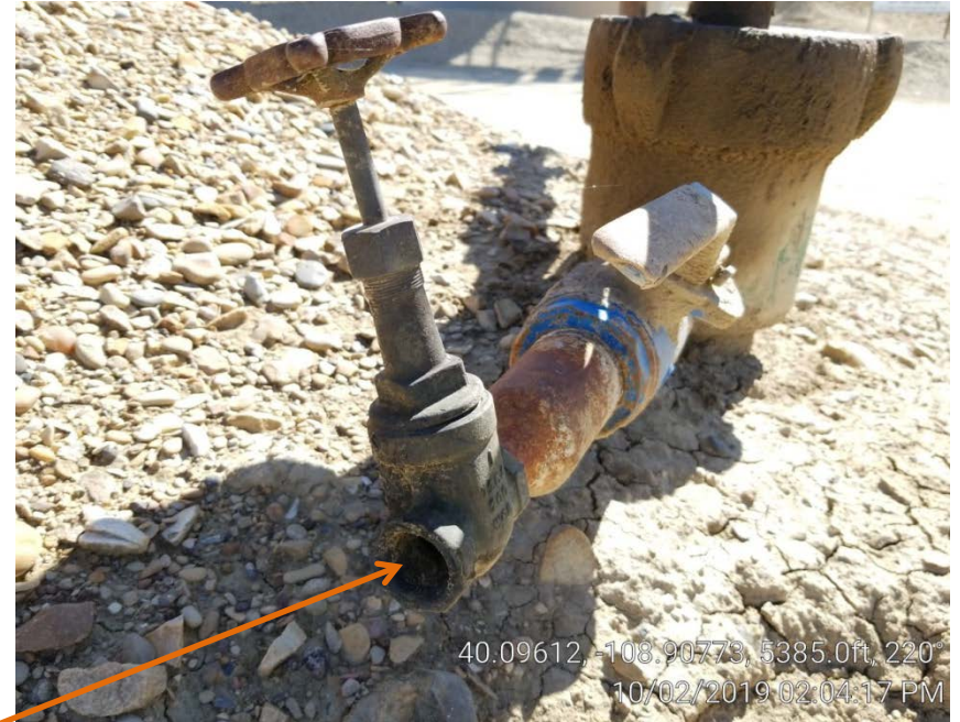
Photo 5. Casing valve.
